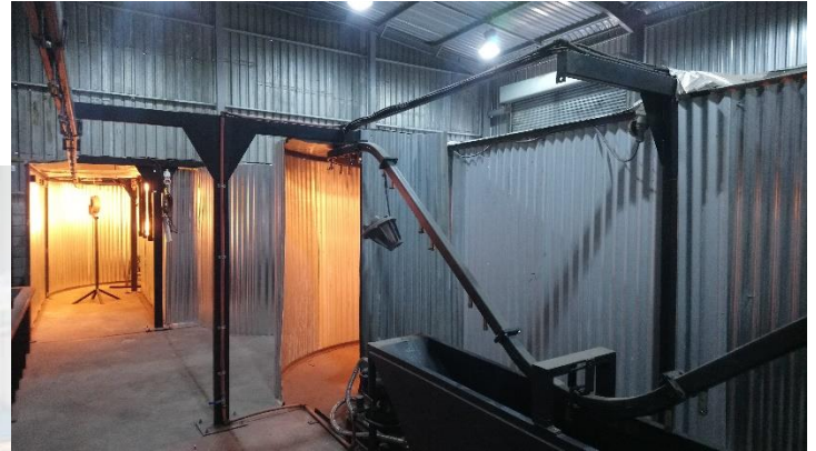
Dipping plant track
