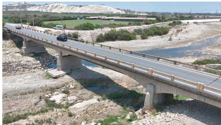
Figure 9. Puente Huamani Bridge in Pisco, Peru.
