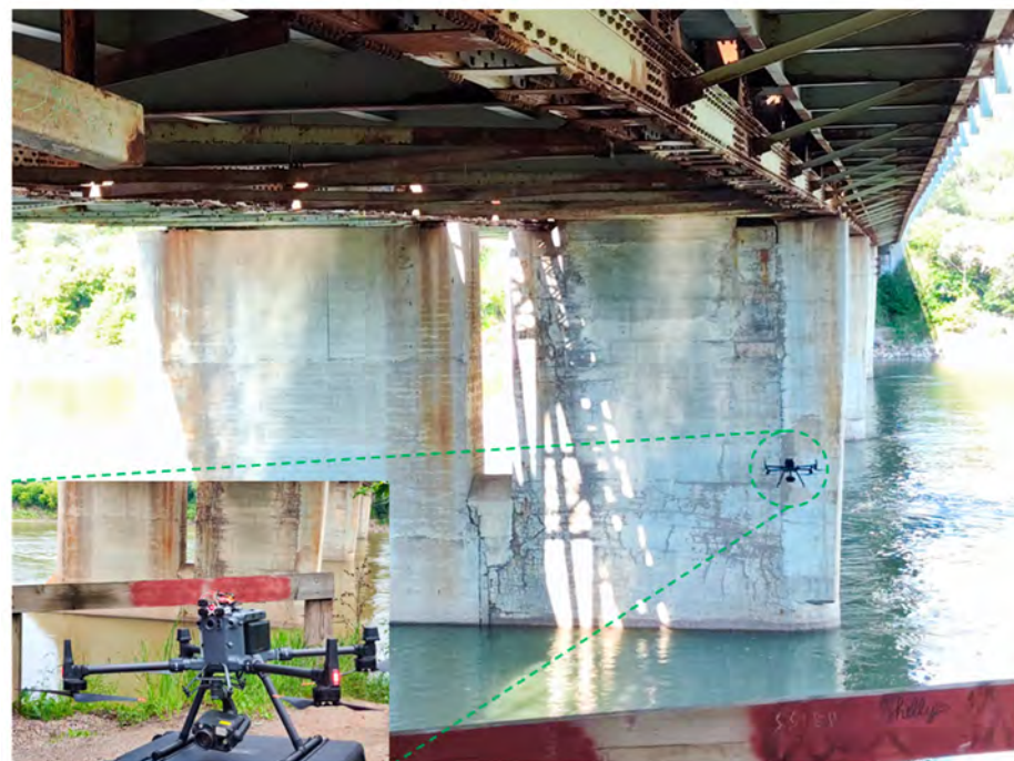
Figure 11. Cross-platform field deployment at the Low Level Bridge in Edmonton, Canada, using the DJI Matrice 350 RTK carrying the same metrology payload.
