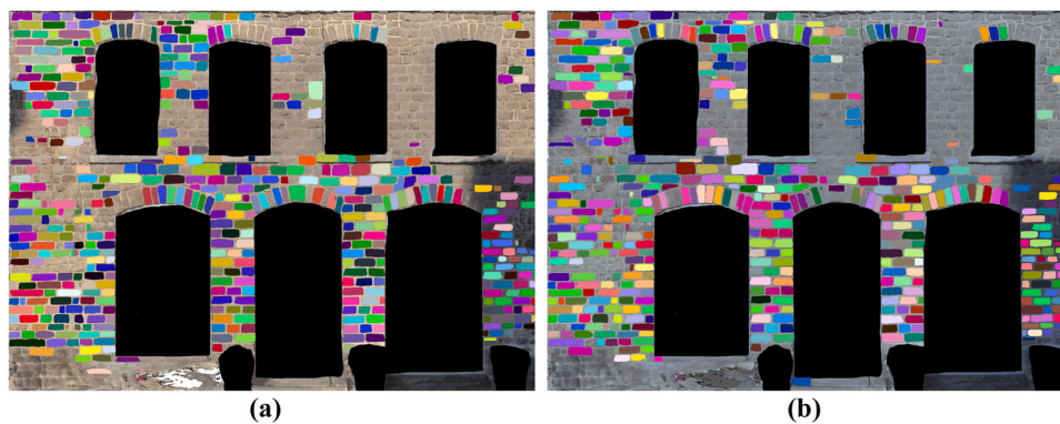
Fig. 6. Southwestern façade masks: (a) no color grading - raw output and (b) color grading - raw output.
