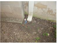
Extend down spouts 3 feet from foundation perimeter or install splash blocks.
