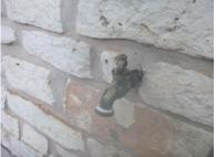
Back flow prevention is missing at exterior hose bibbs. Protective sleeves and collars are not present or damaged at exterior hose bibb masonry veneer penetrations. The hose bibbs drip when operating.
