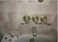
The bathtub hot water valves do not have an identifiable temperature limiting device as currently required by local and National Building Codes.
