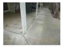
The rear porch posts lack offsets from the concrete patio to prevent water damage.
