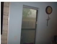
Various windows were observed to have moisture or staining between double panes. This is the result of failure of the seals between double panes allowing moisture to enter space and causes "fogging" to windows.
