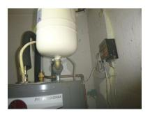
The garage water heater lacks a required electrical disconnect.
