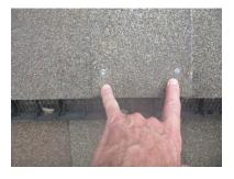
Seal all exposed fasteners to prevent possible water penetration at flashings, roof penetrations, satellite dishes, etc.
