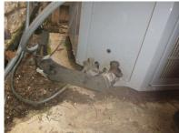
The refrigerant lines are not adequately protected from damage. Protective sleeves are required to prevent abrasion damage, UV exposure, and potential leakage. [IRC N1103.1.1] [R403.4.1]
