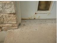
The exterior door off the garage is subject to water damage due to the close proximity of the adjacent deck or patio slab from back splashing and exposure. Storm doors are very effective at protecting exposed exterior doors from damage. Water damage was noted to the door and adjacent areas.
