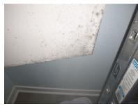
There is excessive moisture and biologic growth at the HVAC enclosures in the garage and upper hallway. -Some biologic growth can be harmful.
