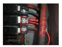
Double tapped breaker present. Manufacturer specifically forbids attachment of more than one branch circuit wire to each breaker.
