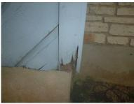
Siding and trim on the chimney is water damaged, has large open gaps, holes, loose trim, and damaged Weather Resistant Barriers (WRB).
