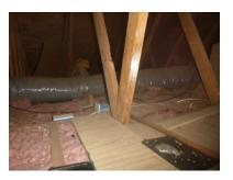
Insulation is minimal by current requirements. Energy efficiency of structure can be greatly increased with additional insulation coverage. Current energy codes require a minimum R-38 insulation value (roughly equivalent to 14-16" of loose fill insulation).
