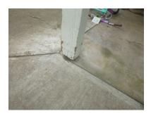
The right side rear porch post is water damaged and is no longer anchored to the patio.
