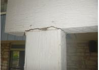
Patio posts are butt jointed and toe nailed.
