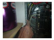
Drywall gaps around the panel are greater than the allowed 1/8". [NEC 312.4] -Seal the gaps.
