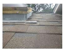
Secure all lifting flashings flush to the roof surface.
