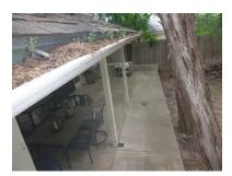
Clean out gutters, reseal joints as necessary, level for drainage, and extend down spouts 3 feet from the foundation perimeter and/or install splash blocks.
