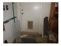
Interior garage door is not fire rated for location installed due to a pet door. Interior garage doors are required to be 1 3/8" solid core/metal [IRC R302.5.1].
