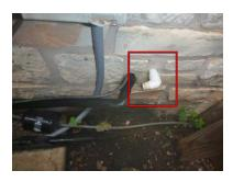
Extend the A/C condensation drain line(s) at least 3 feet from the foundation perimeter.
