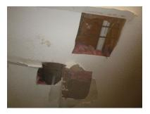
Leakage has caused water damage to the garage ceiling.
