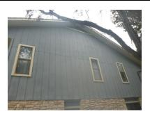
Head flashing is not present <u>above the projecting exterior wall trim</u> at the windows and doors as required. Head flashing is required to prevent bulk water penetration of the exterior wall assemblies at these vulnerable areas and to protect the trim from exposure and water damage. [IRC R703.4(4)]
