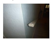
Hand rails terminate improperly. Hand rails are required to turn back at the adjacent wall plane to avoid
