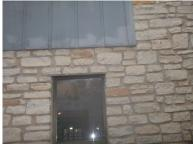
Weep holes are missing over the window and/or door lintels.
