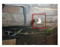
Extend the condensation drain line(s) a minimum of 3 feet away from foundation perimeter to avoid excessive deposit of water directly adjacent to foundation perimeter.
