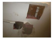
Plumbing in the garage ceiling is exposed and subject to freeze damage in extreme weather conditions.
