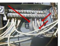
The Grounded (bare copper wires) and Grounding (white/neutrals) are bonded at the Sub Panel. This is never allowed at Sub Panels as it creates a false, or circular ground path. Grounded and Grounding conductors are to be bonded ONLY at the Service Disconnect Panel. [NEC 480.40] Safety Hazard.
