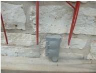
Replace the exposed exterior receptacle cover(s) with a wet location rated, "in use", "bubble cover". [NEC 406.9(2)]
