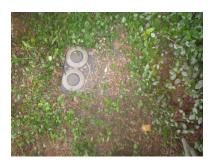
There is no home owner's cut off valve. System cut off is at city side of the water meter.
