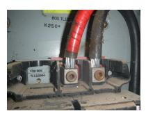
The aluminum feeder wire terminations lack the required application of anti oxidation paste.
