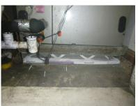
The air filters are dirty, damaged, and past due for change out.
