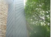
Trim trees back a minimum of 3 feet from the roof surface to avoid abrasion damage of the roof surface.
