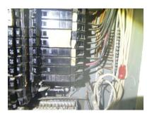
The multi wire circuit(s) lack required trip ties. [NEC 210.4].
