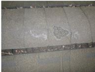
A number of areas have damaged and missing shingles from tree abrasion.
