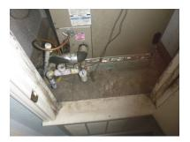
Wall trim and enclosure platforms at the HVAC enclosures are water damaged.
