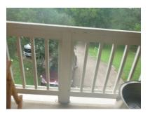
Stair and guard rail spacing will allow passage of a 4" sphere. This is considered a safety hazard. [IRC R312.3]
