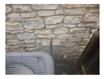
The HVAC disconnect(s) lack required clearance(s) for access. [NEC 110.26(A)]
