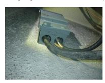
Wire clamps are missing at the wiring entrances to the upper level HVAC air handler disconnect. This may allow damage to the conductor insulation which could result in an electrical fault and become a shock/fire hazard. Missing cable clamps and bushings are considered to be a latent fire and safety hazard. [NEC 300.4(B)(1)]
