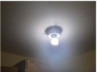
Install protective cages or globes on all exposed attic and closet lights to prevent physical damage. -Several fixtures have missing covers, cages, and globes.
