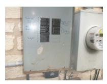
Overhead Feeder. Al SEC. Cu BCW. 7 throws required for system disconnect (max. 6 allowed).
