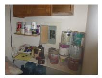
Panel lacks required clearance for service access (30"x36"x78") [NEC 110.26] -Shelving blocks required access.
