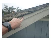
Drip and rake edge flashing is not present where currently required. [IRC R905.2.8.5]
