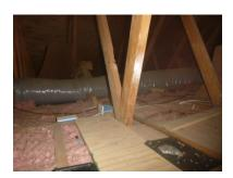
Grey flexible ducting observed. Ducting of this type is known to have a higher than normal failure rate due to the lack of resistance to UV radiation in attics. Some ducts were observed to have degraded vapor barriers which is a sign of failure. Recommend budgeting for replacement.
