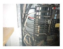
Breaker(s) have a "white" wire utilized as a "hot" conductor on one leg of the circuit without being designated as such. For example, this white wire should have a piece of red tape wrapped around it to designate it as a "hot" conductor versus a "neutral" conductor. [NEC 210.5]
