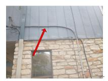
The SEC cables are exposed. Currently, code requires SEC cables to be contained within approved and listed raceways.
