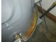
The expansion tank is corroded and actively leaking down the unit and into the drip pan.
