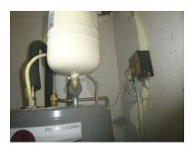
The water heater lacks a required electrical disconnect. [NEC 422.30]
