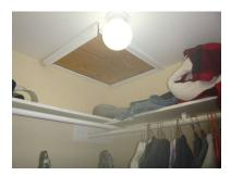
The attic lacks proper provisions for access. The attic access shall be no less than 30" x 22" when in a ceiling or wall. The attic access shall be in a hallway or other *readily accessible* location. Unobstructed headroom clearance above the access shall be a minimum 30". [IRC R807.1]
