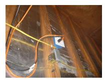
Extension cords are present in the attic. If wiring penetrates any walls, structures or enclosures, or runs through attic it is considered a fire hazard. Extension cords should not be used for permanent appliances or as a substitute for structure wiring. [NEC 400.8 (1)]
