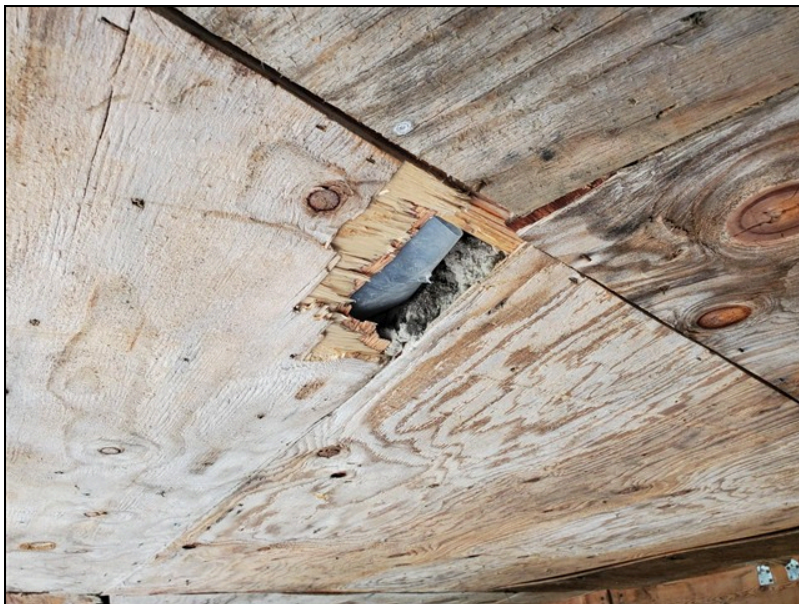
8.1 Item 1(Picture) gap in plywood sheathing below sunroom
