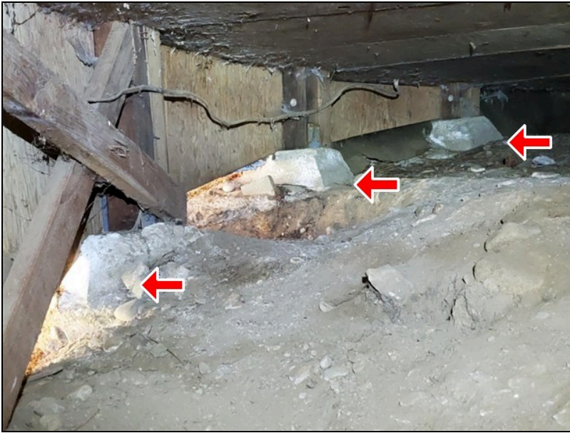
4.2 Item 4(Picture) piers
