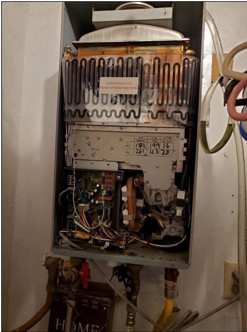
5.2 Item 4(Picture) Interior view
