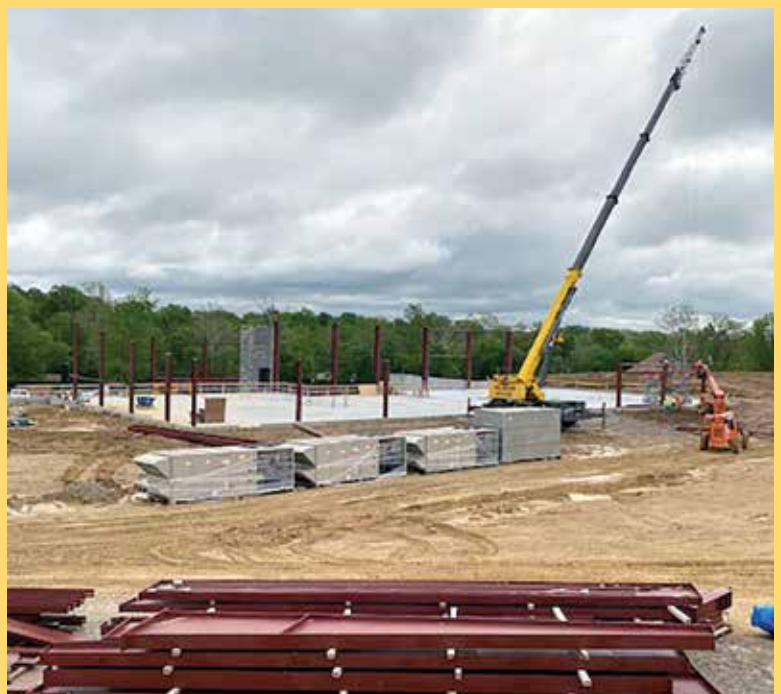
Erlinger Crane - Fulton Community Center - Shane Hale - operator.
