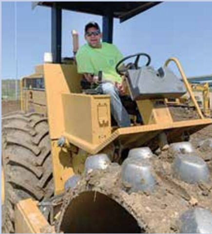
Todd Rundel running a roller for KCI at 44270 interchange .
