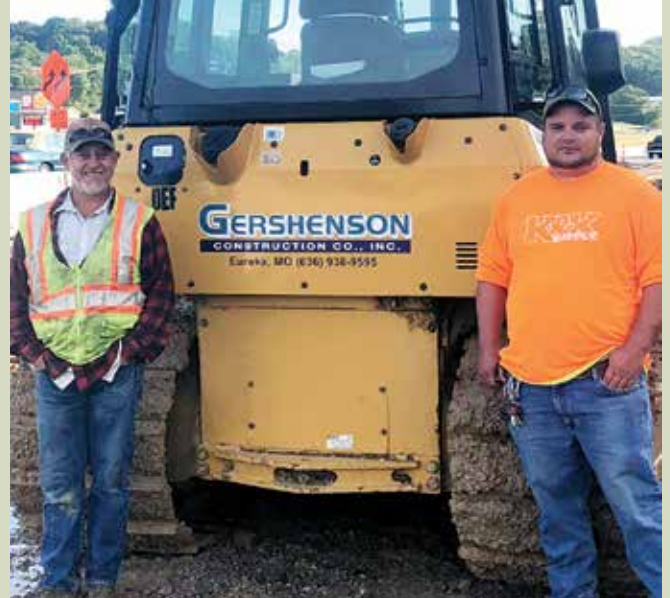
Mathew Gegg and Bradley Kawelaske working for Gershenson Construction at the MODot bridge replacement on Hwy over Saline Creek.
