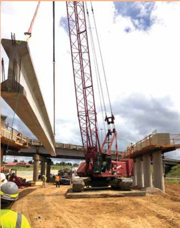
Garrett Moll setting bridge girders at Center Junction in Jackson, Mo.
