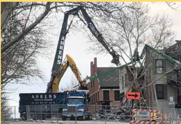
TJ Ahrens Excavating - High Street Demolition – Jefferson City.
