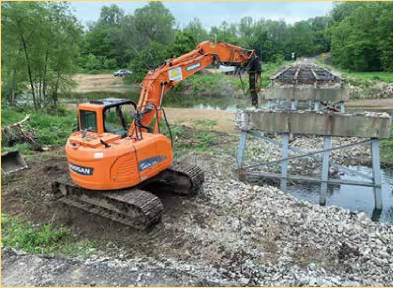
Don Schnieders Excavating – Hwy A bridge – Gasconade County – Shay Frank, Operator.
