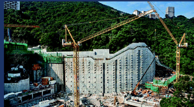
Permanent tie-back at development site at Stubbs Road
