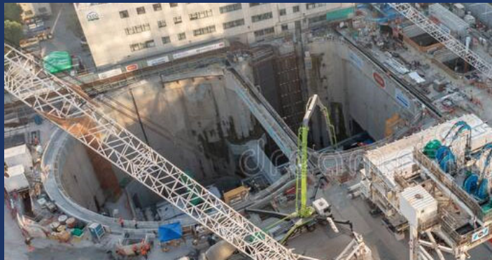
Trunk Road T2 (2022)
