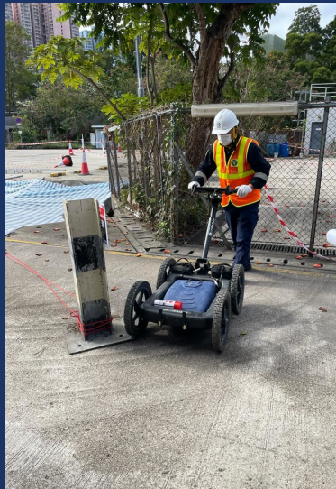
Ground penetration radar
