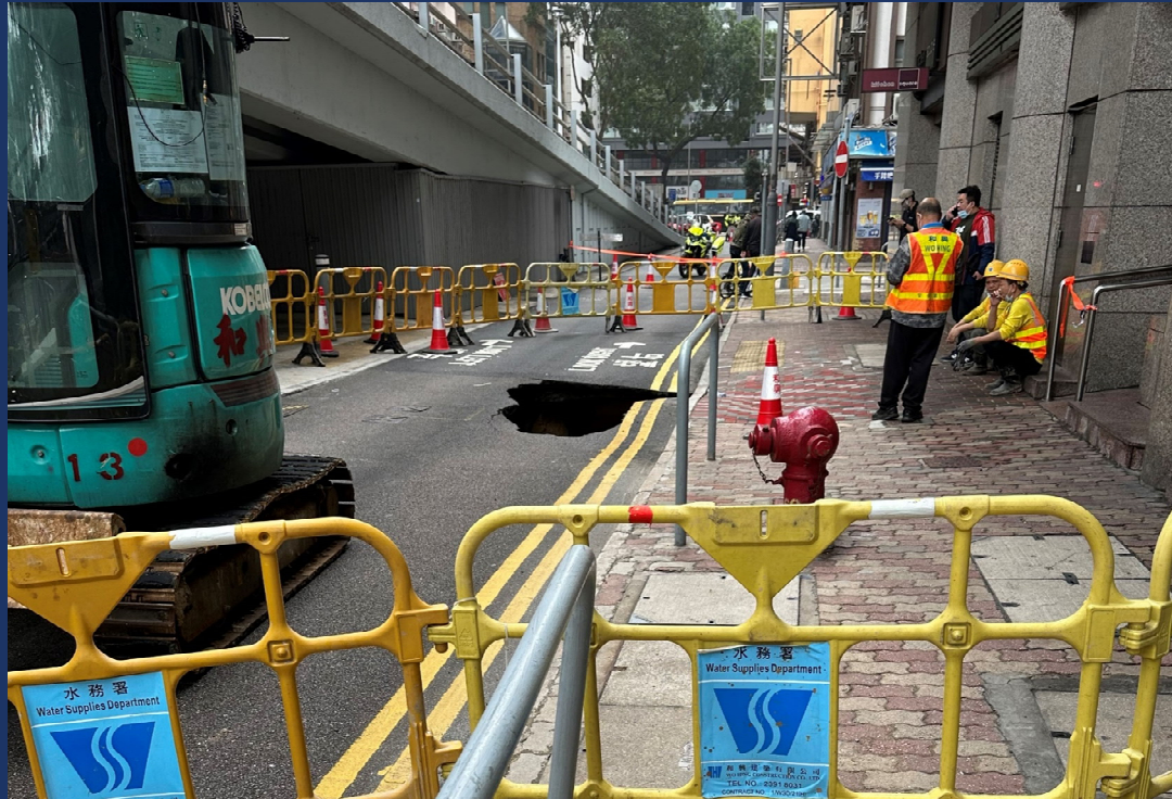
Emergency repair for burst water carrying services
