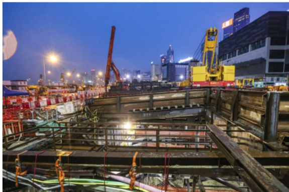
Public safety has to be assured following the disclosure by rail giant MTR that 131 locations on troubled Sha Tin-Central link require follow-up action. Photo: Felix Wong
