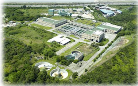
Water treatment works
