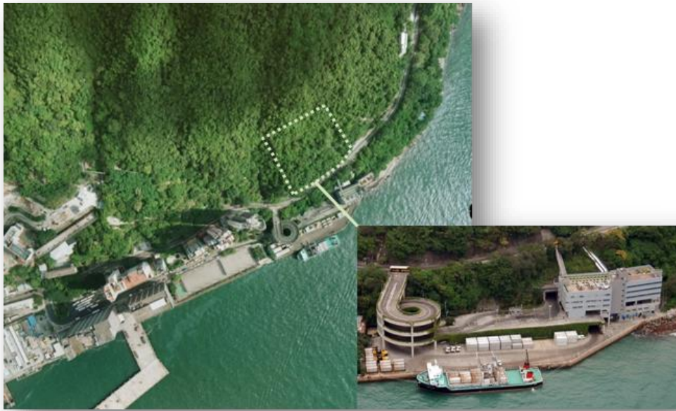
Island West Transfer Station
