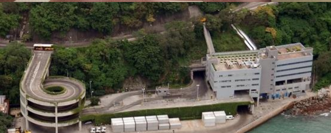
Island West Transfer Station (1997)
