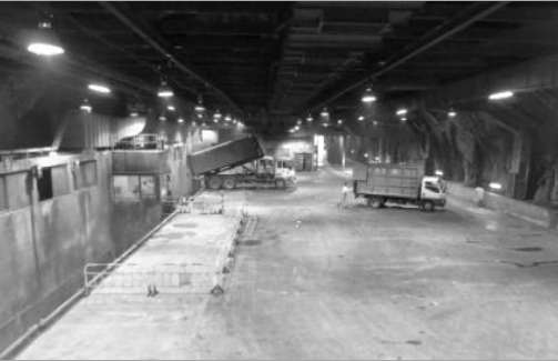
Refuse Transfer Station
