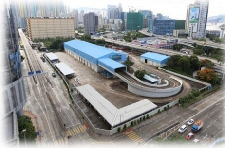
Refuse transfer stations
