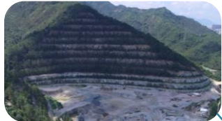
Lam Tei Underground Quarry (Upcoming IDC Study)
