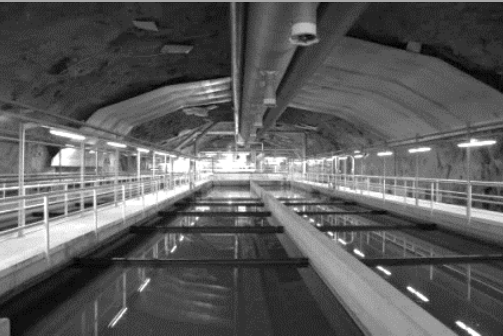
Sewage Treatment Works
