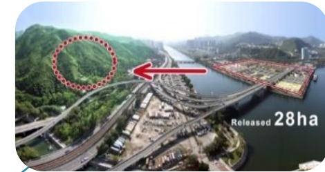
Relocation of Sha Tin Sewage Treatment Works (Construction)
