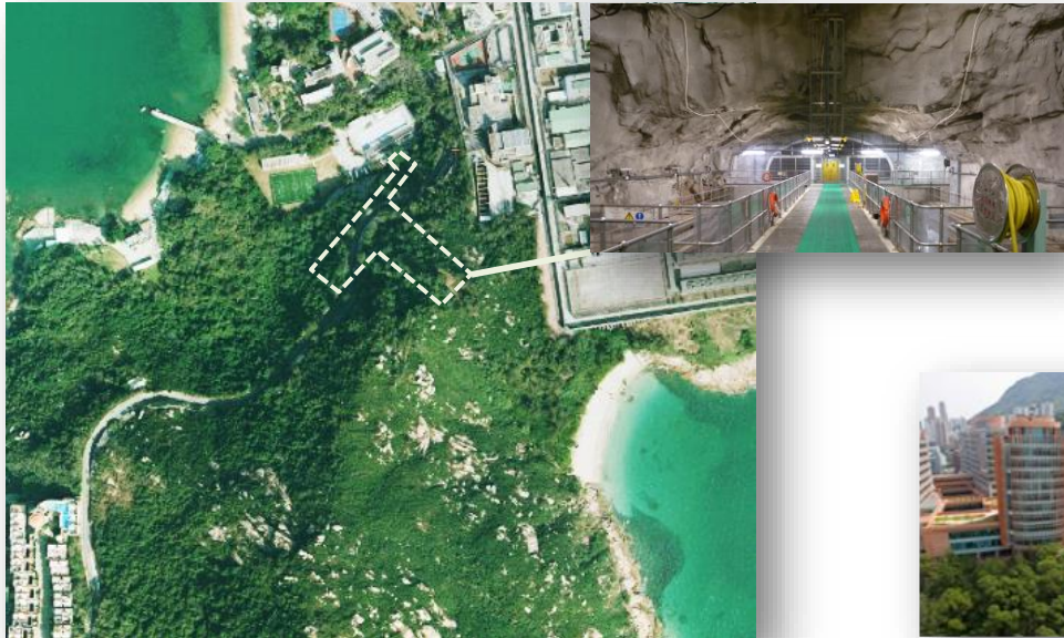
Stanley Sewage Treatment Works
