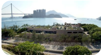
Relocation of Sham Tseng Sewage Treatment Works
