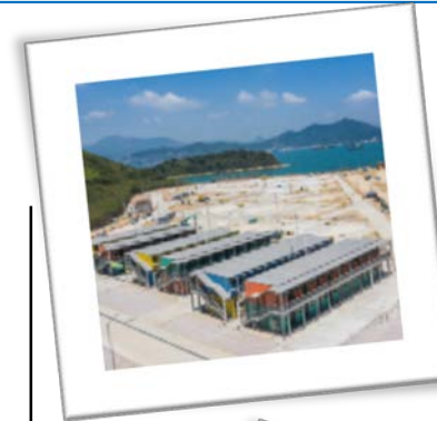
Quarantine Camp in Penny Bay – Phase 1A 110 units built in 56 day
