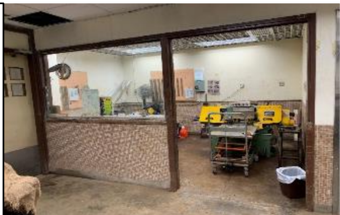
Aging facilities and inefficient design
