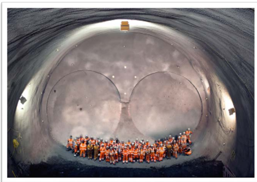
Crossrail – Stepney Green junction’s Eastbound SCL cavern
