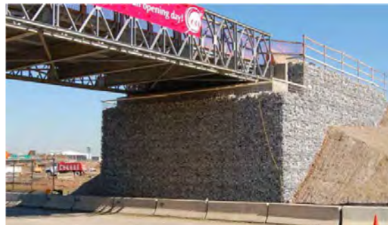
Figure 8: TerraTrel Reinforced Earth True Abutment
