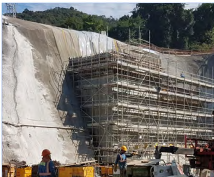
Plate 3: Construction of goose-shaped wall in progress
