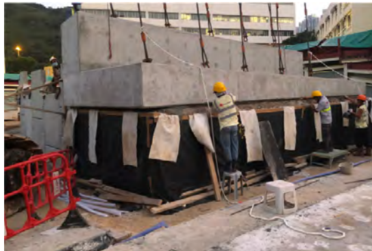
Figure 4g: Erection of the precast L-shaped R.C. seating
