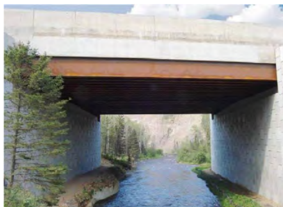
Figure 6: Suncor Steepbank River Bridge
