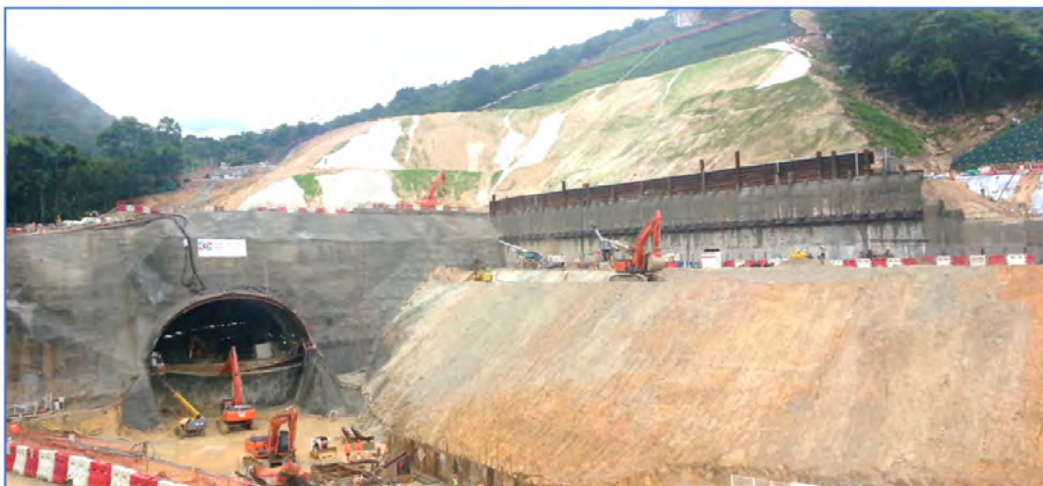
Plate 2: Southbound tunnel at the Northern Portal in phase with construction of the soldier pile wall
