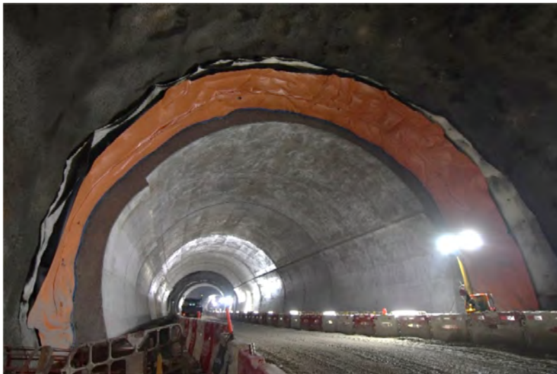
Figure 4: Conventional Cast-in-situ Permanent Concrete Lining
