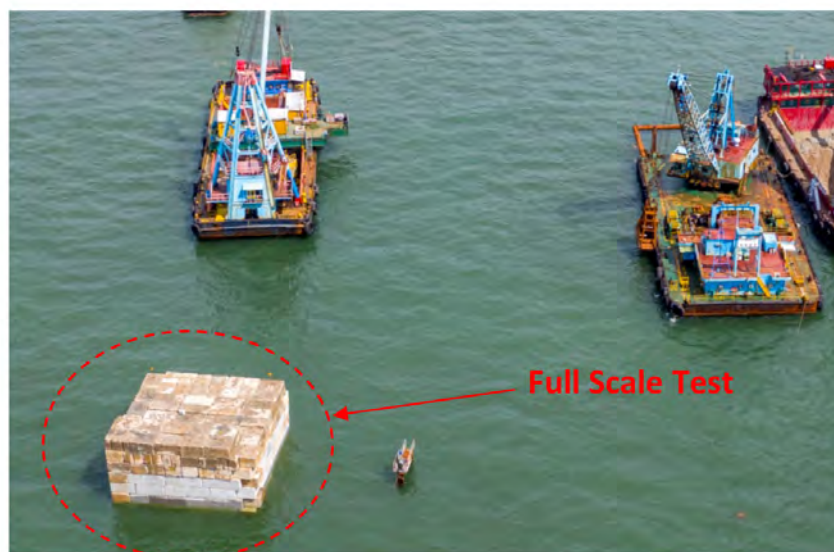
Plate 1: Site Photo of loading concrete blocks
