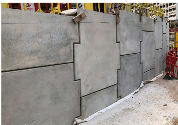
Figure 4h: Completion of Reinforced Earth wall
