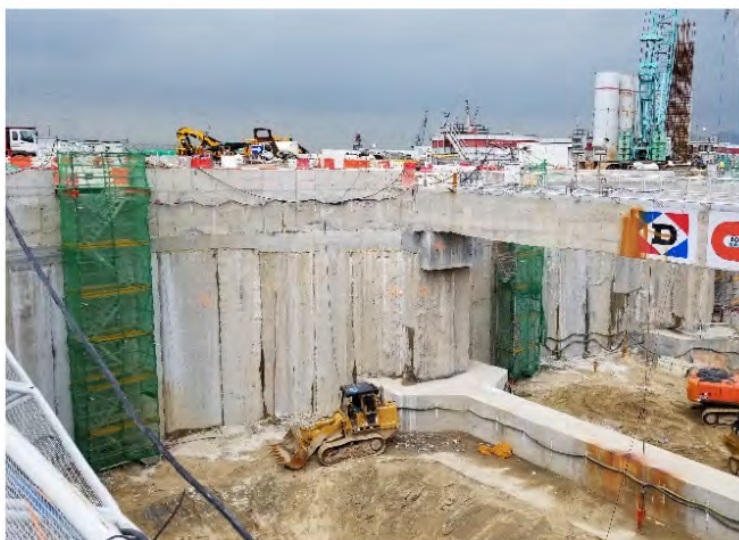
Plate 1 – Exposed Y-Panel with Struts and Arch Cells
