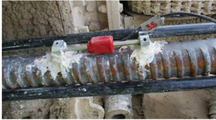
Plate 5: Strain gauge installed on a tie-back
