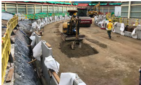
Figure 4d: Placing selected backfill
