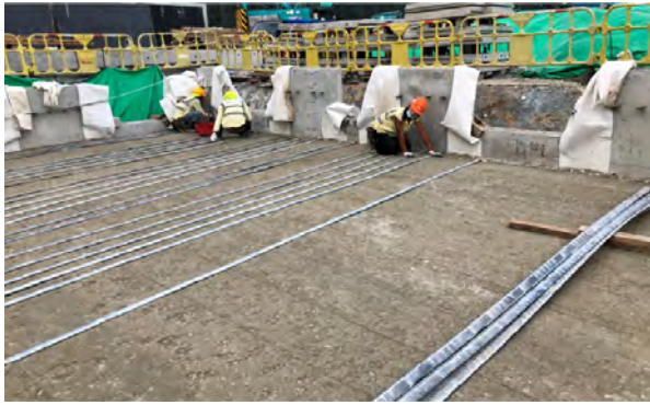
Figure 4e: Placing reinforcing strip
