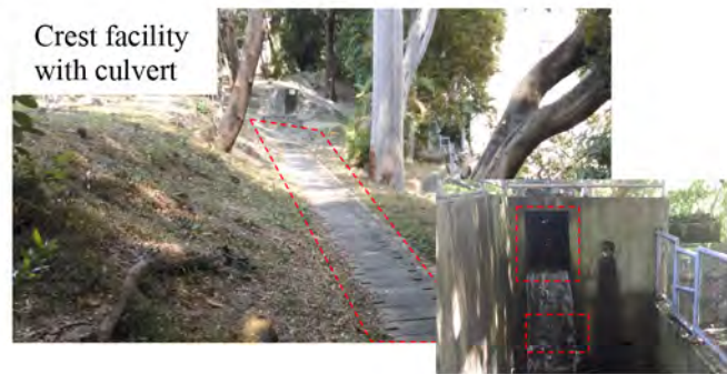
Plate 2: Crest facility at the study feature
