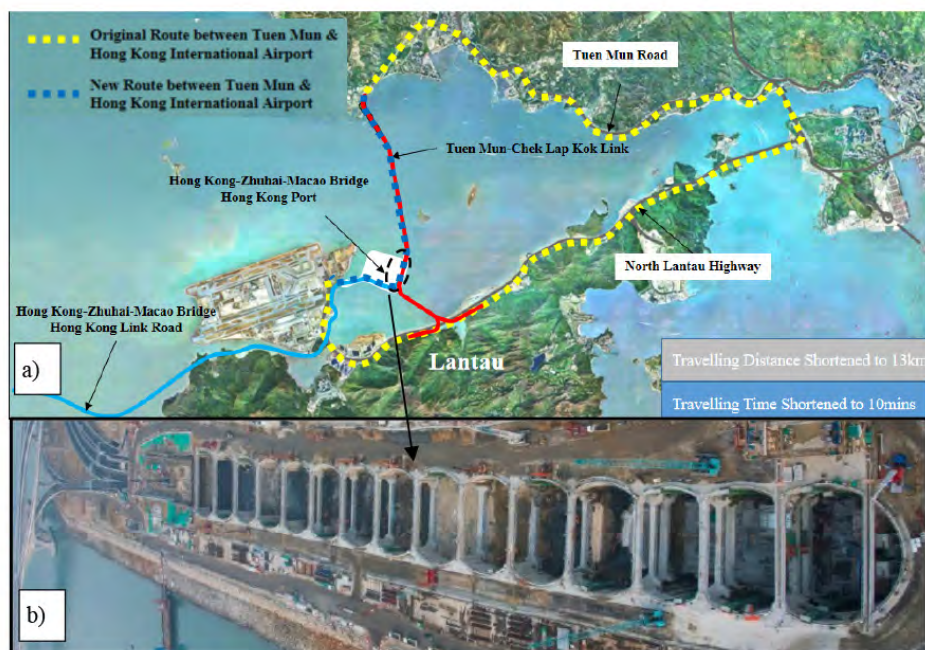
Figure 1: a) Tuen Mun Chek Lap Kok Link Project Location, adapted from www.hzmb.hk/eng/about_tmclkl.html (Accessed on the 31/03/2021); b) Hybrid ELS Scheme, courtesy of Dragages Bouygues Travaux Public JV
