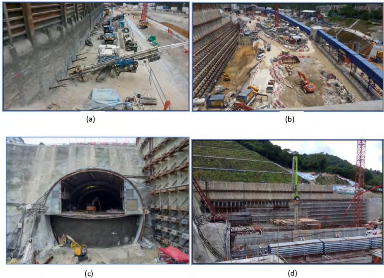
Plate 4: Construction of composite retaining wall at Northern Portal
