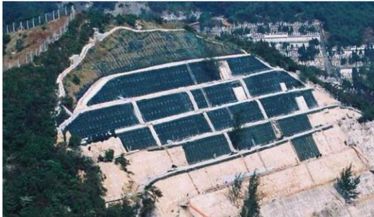
Site Formation Work (e.g. slope stabilization, retaining structures)
