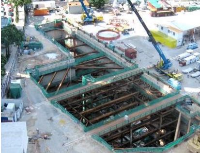
Excavation & Lateral Support Works
