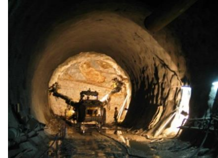
Tunneling works (e.g. Tunnels, caverns, shafts)
