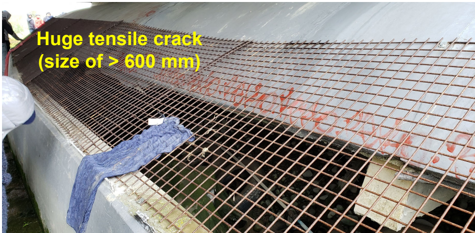
Another persistent crack at a pathway below the bridge deck
