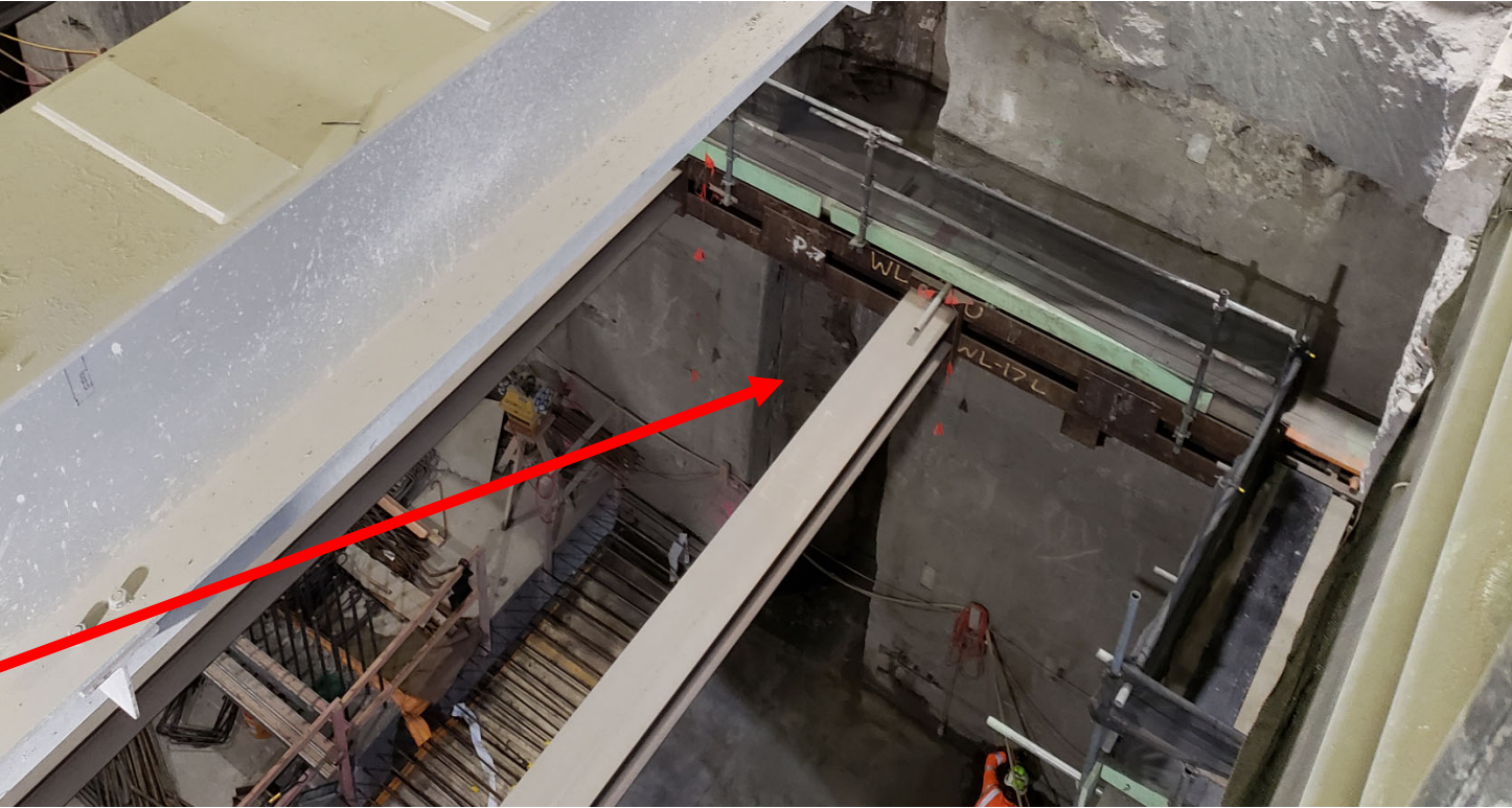
Jet grouted column among diaphragm wall panels
