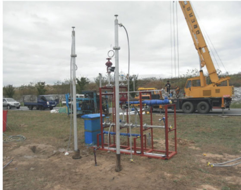
Installed freezing pipe (using liquid nitrogen)
