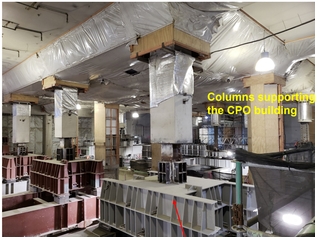
Hydraulic load cell and support frame
