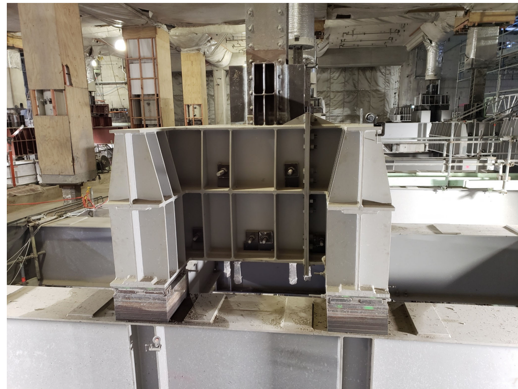
A close-up of the supporting frame
