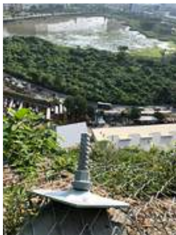
Plate 8: Installation of hot dip galvanized threadbar kit, Ø32mm, grade B500B, rockbolt application in Macao (DYWIDAG Archive)
