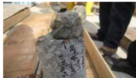
(b) Drilling Break and Irregular Bell-Shaped in Concrete Core
