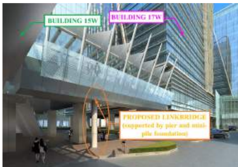
Plate 1: Architectural Picture of the New Linkbridge
