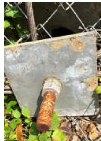
Plate 9: Exposed soil nail head without angle compensation, severe signs of corrosion (DYWIDAG Archive)
