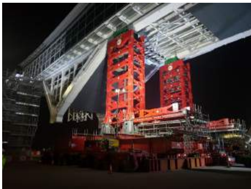
Figure 3: Jacking up of tower supports to raise the Arch Truss
