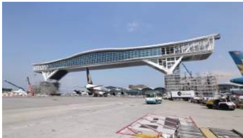
Figure 5: A photograph of Arch Truss after installation
