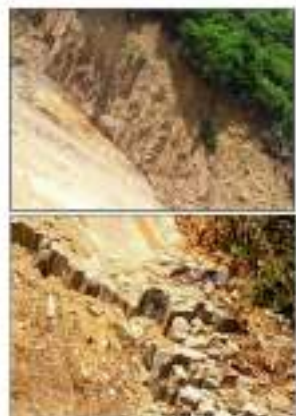
Figure 8: Photos taken by UAV after the landslide
