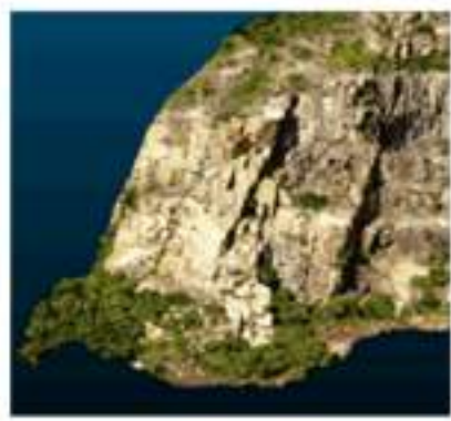
Figure 10a: Overview of rock slope portion generated from UAV photogrammetry
