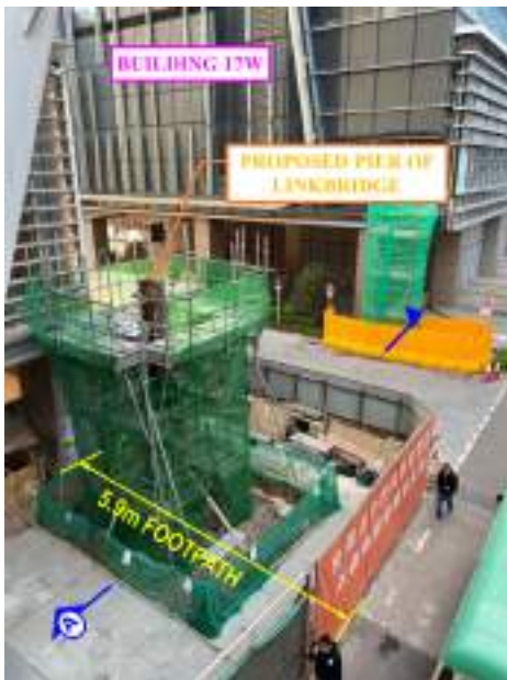
Plate 2: General Site Condition of the Proposed Foundation Works
