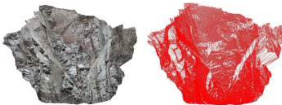
Figure 1: The use of UAV and photogrammetry for slope inspection.
