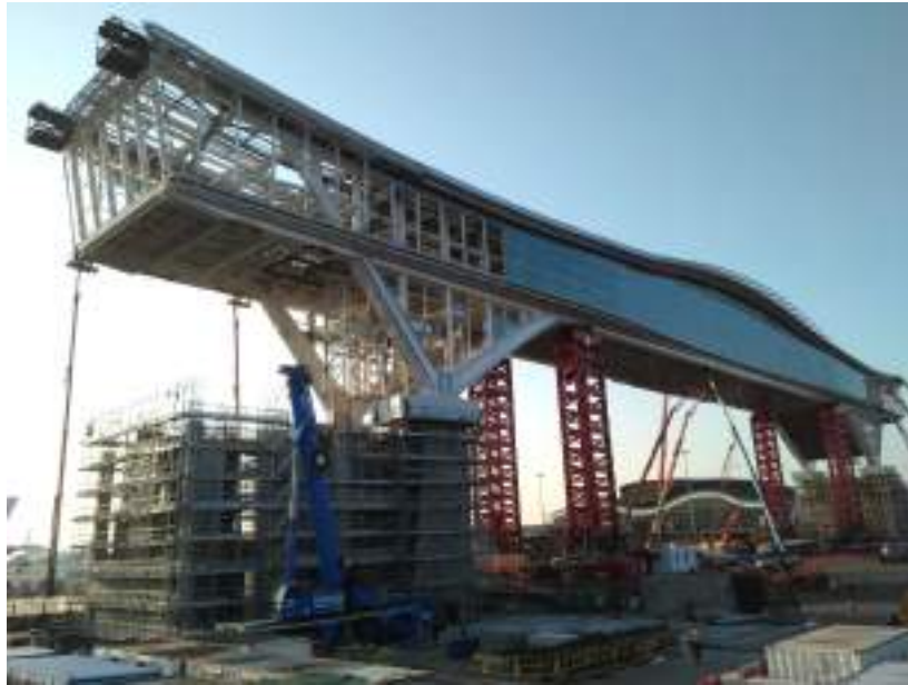
Figure 4: Arch Truss placed in its final position
