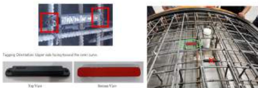
Plate 3.3: RFID Tags (Cast-in) Installation to Precast Segment
