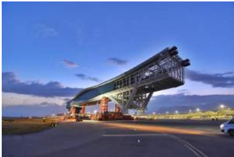
Figure 2: Transportation of the Arch Truss to the location of Main Bridge
