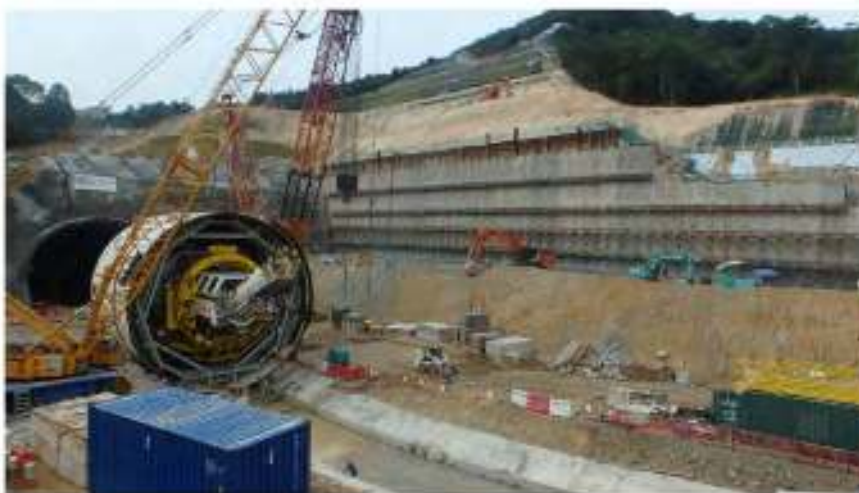
Figure 6: The north portal of the Liantang Heung Yuen Wai Tunnel
