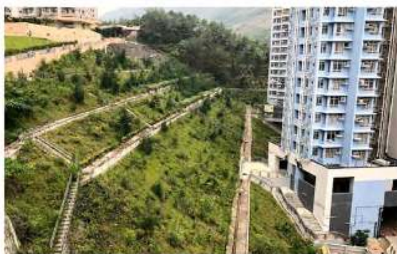
Figure 5: General view on the greening of soil cement slope (photo taken in Aug 2018, about 3 years after plantation)
