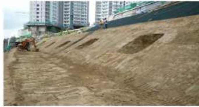
Figure 3: Tree pits of 2m x 2m x app. 1m deep at 8m spacing staggered in rows on the slope
