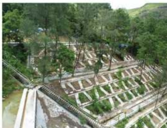
Figure 8: Close look at the free-style grillage beam system on the soil-nailed slope portion with existing trees
