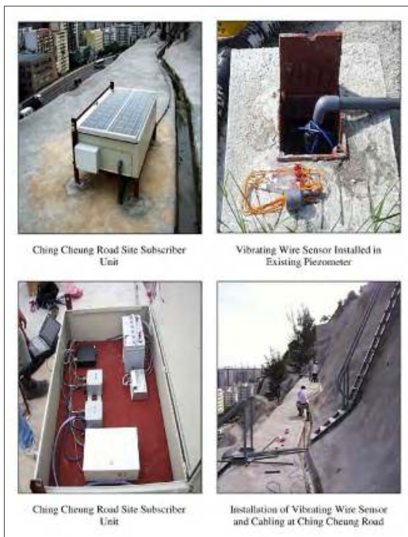
Plate 1: Ching Cheung Road site equipment and setup
