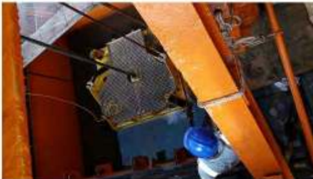
Figure 12: Placement through the Barge Moon Pool
