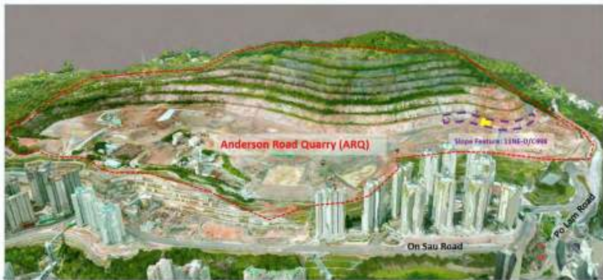
Figure 1: Location of ARQ site and the Slope Feature No. 11NE-D/C998
