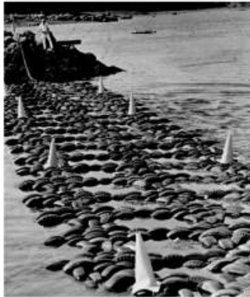
Plate 1: Photograph of recycled tire floating breakwater (Topper Industries Inc.)
