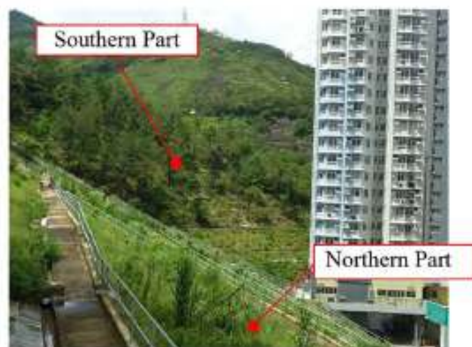
Figure 7: Growth of vegetation on the slope about 2 years after the slope upgrading works
