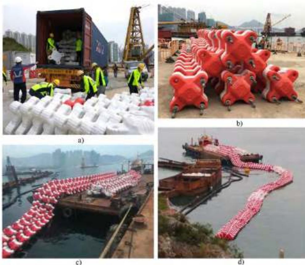
Plate 4: a) Photograph of easy unloading of the floating breakwater units. b) Assembled floating breakwater segment. c) and d) Floating breakwater placement by Flat Top Barge
