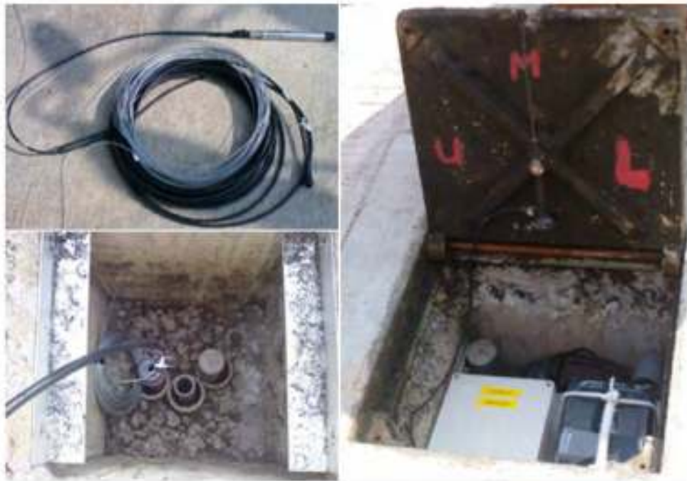
Plate 5: WAGMD installation in a piezometer surface box
