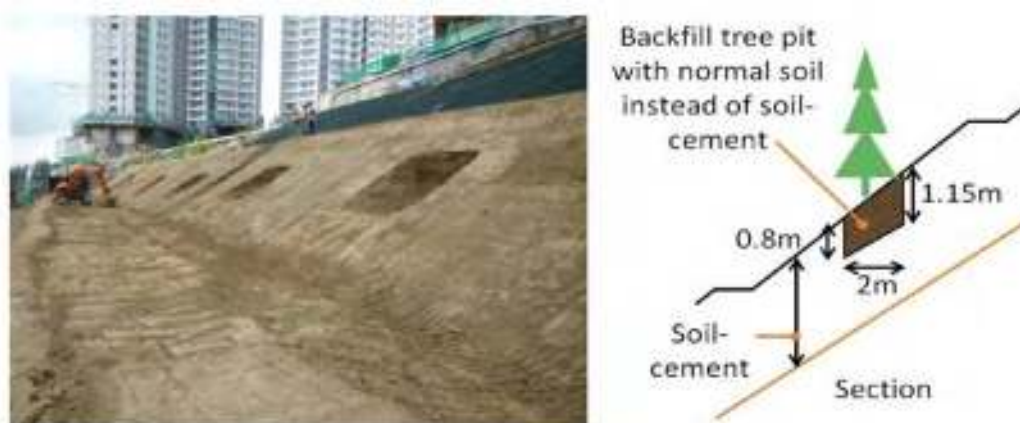
Figure 4: (left) Construction of tree pit in soil cement fill slope & Figure 5: (right) Typical section of tree pit to facilitate slope greening
