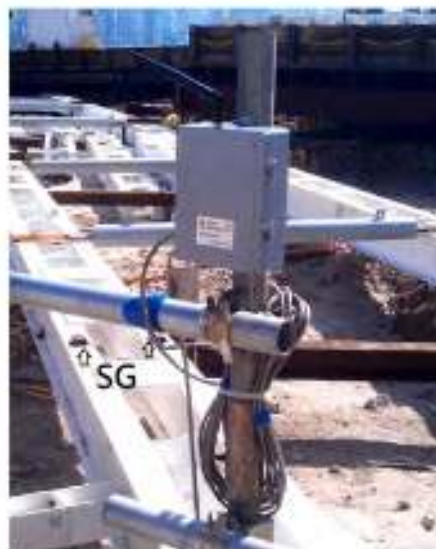
Plate 8: Strut load monitoring using a Wisen 4 channel vibrating wire node
