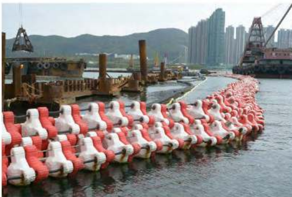
Plate 6: Photograph of installed floating breakwater
