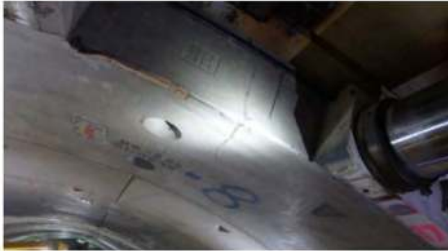
Figure 8b: Cracks on segment (TTR1172)
