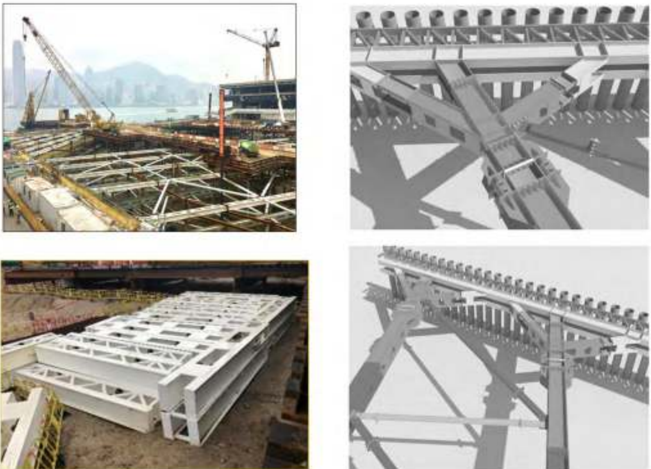
Plate 1: Application of DfMA in shoring modularization
