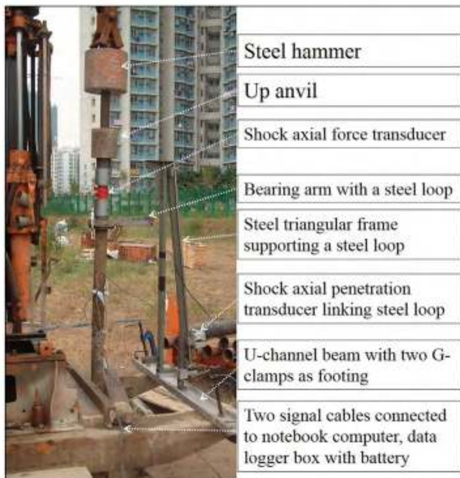
Plate 5: The automatic SPT N-value Monitor in operation at field
