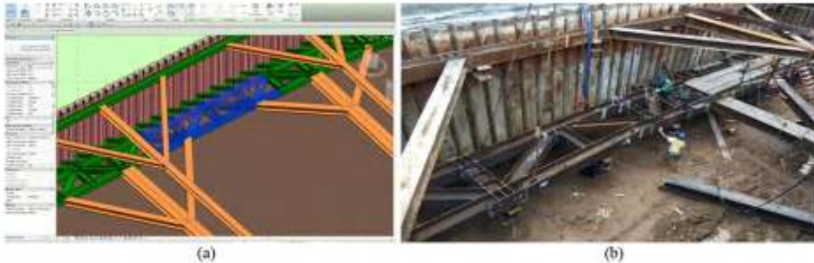
Figure 11: Example of Pre-fabrication Component for ELS Construction
