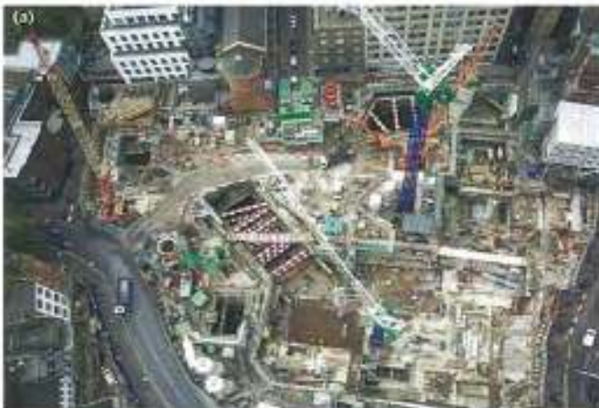
Figure 14: Site photograph of the works (11/12)
