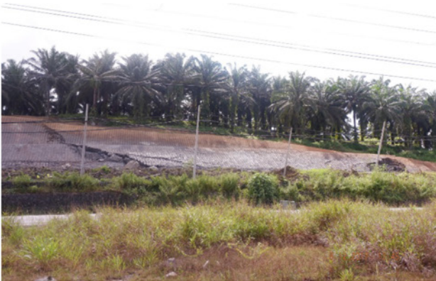
Figure 7: Front view of slope failure in highly and slightly weathered mudstone at Case 3
