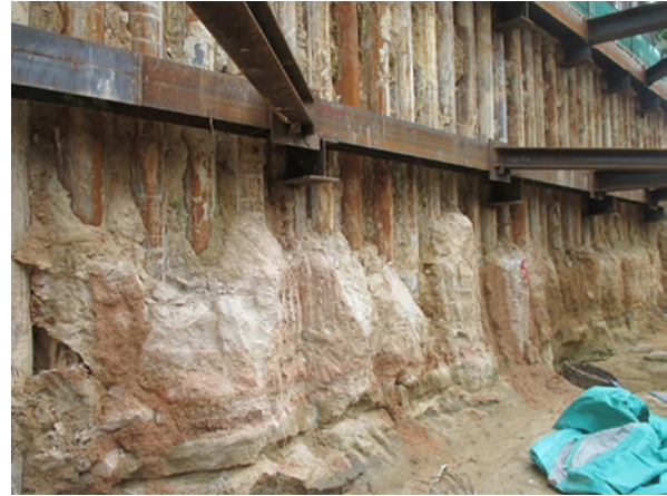
Plate 3: JGC for sealing gaps between pipe piles
