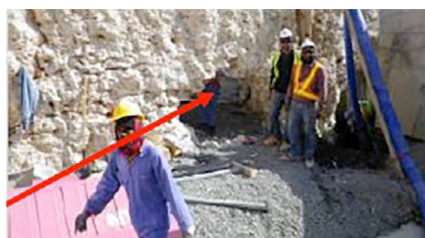
Figures 11 and 12: Karst identified in the Simsima Limestone, immediately above the Midris Shale boundary
