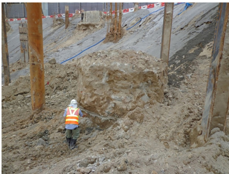
Plate 1: JGC for enhancing stability of temporary cut slope
