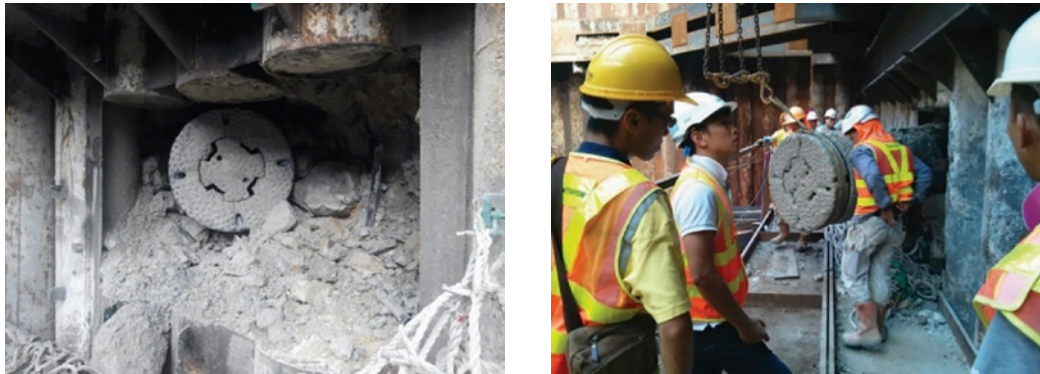
Figure 8: Breakthrough of Canopy Tube with Bohrtec Front Steer System
