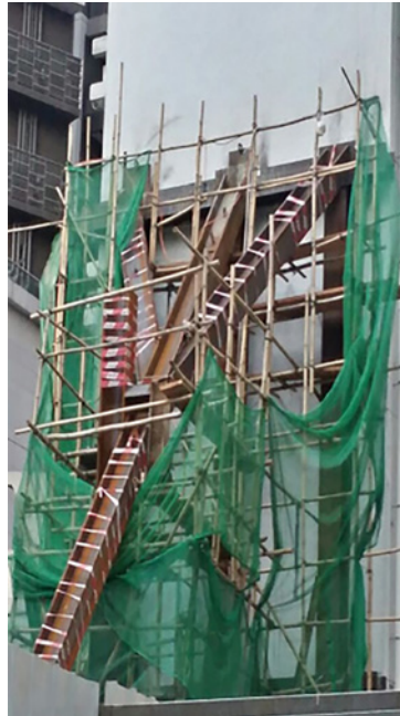
Plate 4: A raking shore supporting a tilted building
