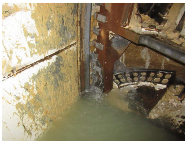
Figure 28: Groundwater pressure increases (Karst)
