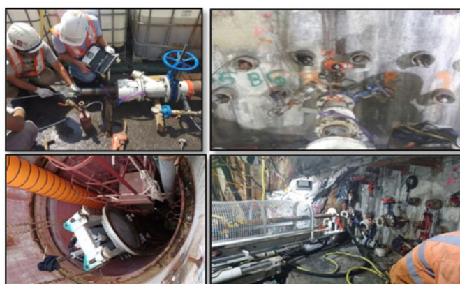
Figure 11: Site photos for horizontal grouting (bentonite or water)
