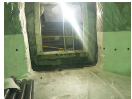
Figure 17: Cross Passage support frame
