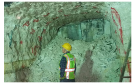
Figures 38: Central span excavation
