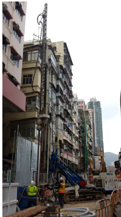
Plate 4: Jet grouting for protecting old building
