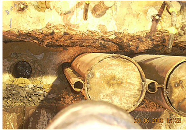
Plate 7: Interlocking pipe piles for a tunnel connection (Courtesy of GCL)
