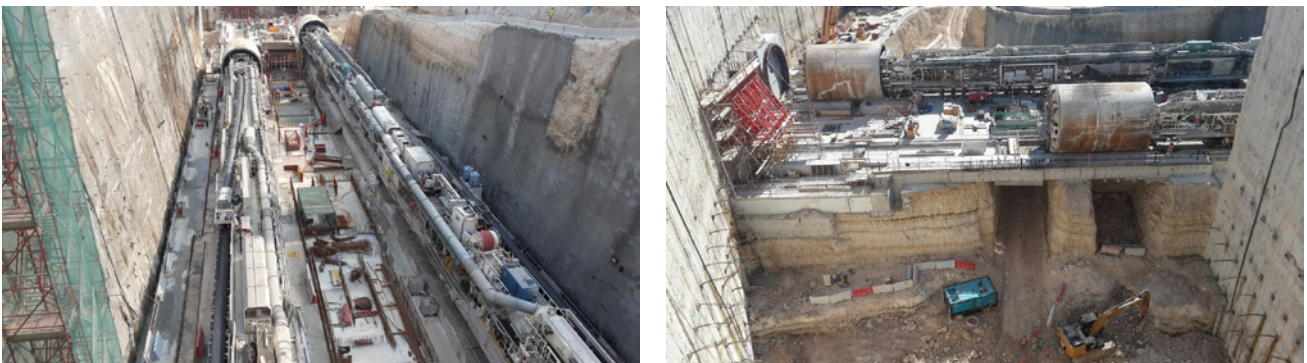
Figures 23 and 24: TBM transfer through Al Saad C-Ring
