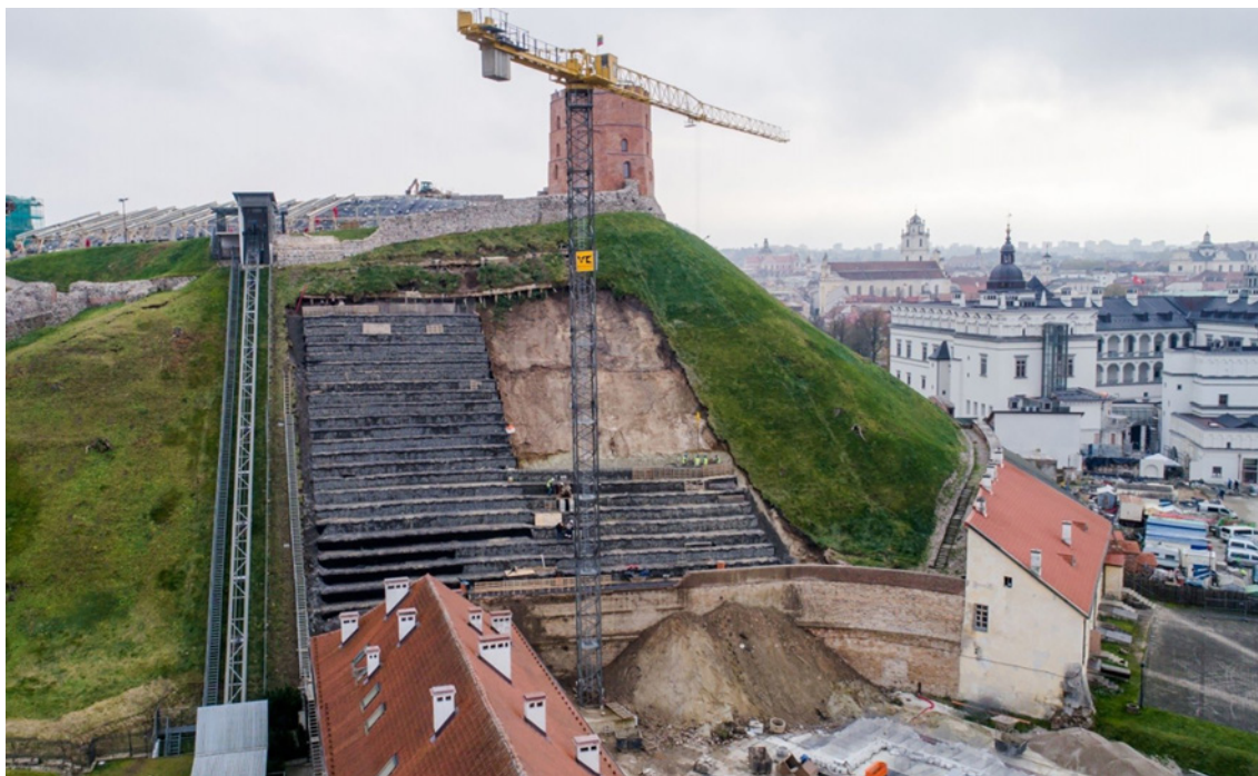
Figure 14: Gediminas Hill north part slope stabilisation with gabions wall installation
