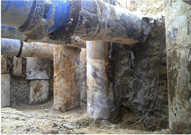
Plate 2: Jet grouting for sealing up utility windows
