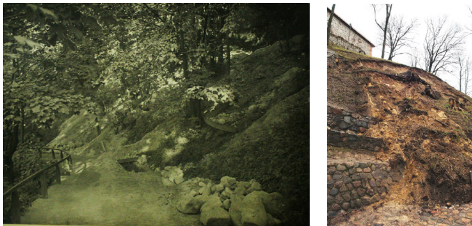
Figure 2: Gediminas Hill slopes instability: on the left had in period of 1930-1938 and on the right hand in period of 2004 and 2008 (Photos from Lithuanian National Culture Heritage Centre archive)
