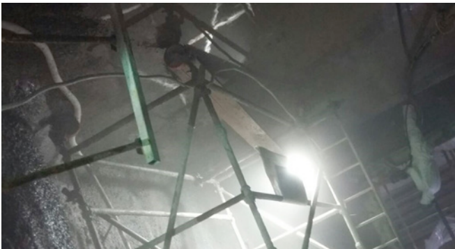
Figures 39 and 40: Waterproofing membrane scaffold erection and placement
