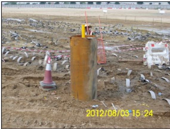
Plate 2: Inclinometer with extendable steel casing
