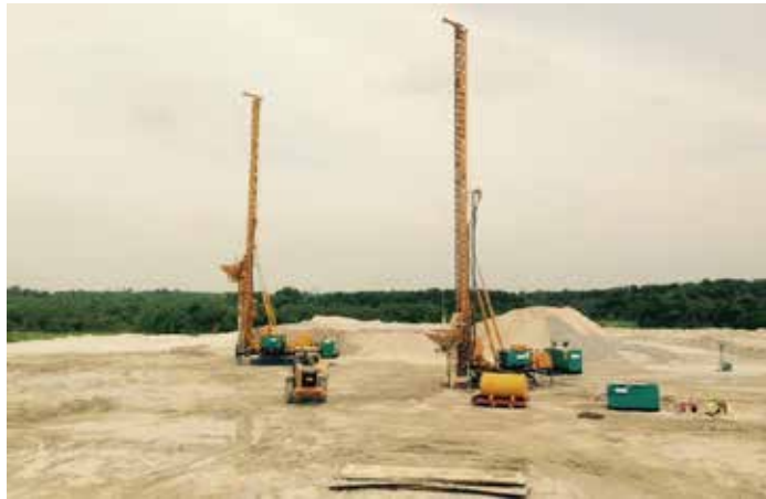
Figure 9: Granular working platform, which will then serve as drainage layer
