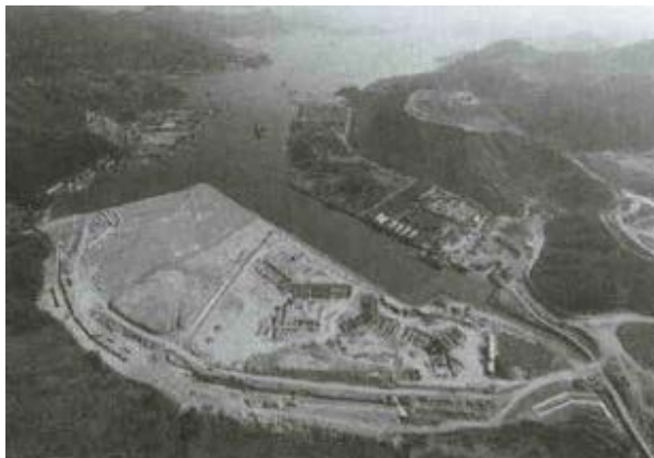
Figure 9: Reclamation works in Tseung Kwan O
