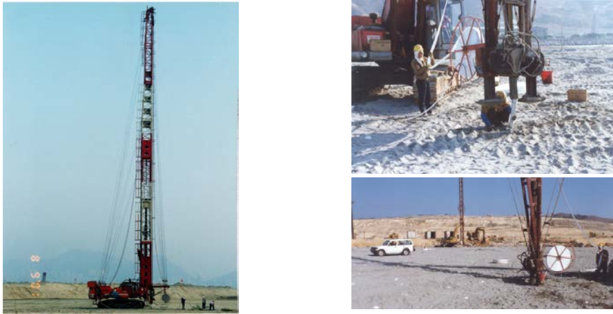
Figure 6: The set-up at the land based PVD installation rig
