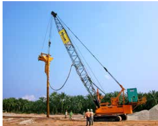
Figure 4: Dry bottom-feed columns installed using the crane hung method, Malaysia, 2006.
