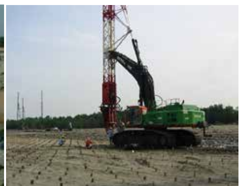
Figure 3: PVD installation
