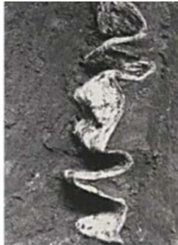
Figure 9: The bent shape of a PVD when subjected to large ground settlements (after Staplefeldt, T.)
