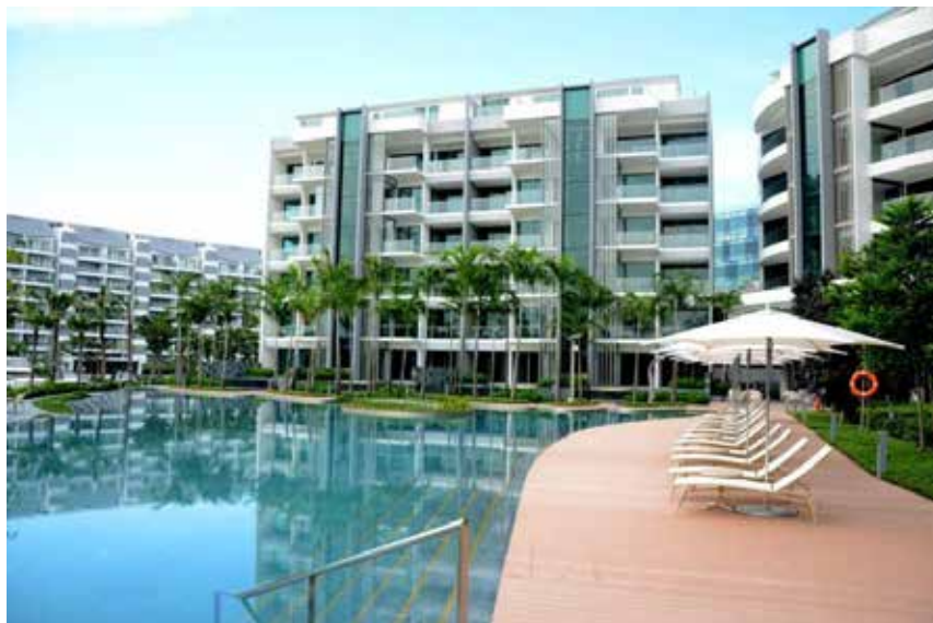
Plate 6: Completed luxury residential building on reclaimed land supported by improved ground without deep foundation (photograph courtesy of Keller Singapore)
