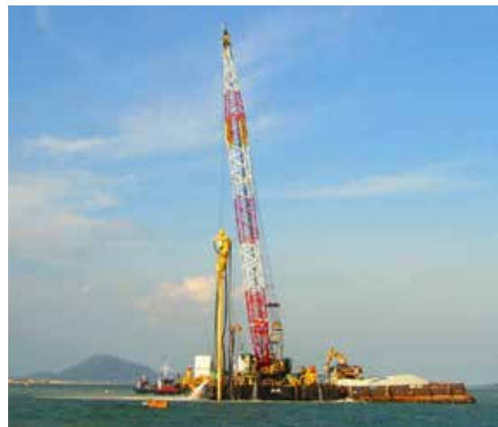
Figure 16: Offshore column installation in progress.
