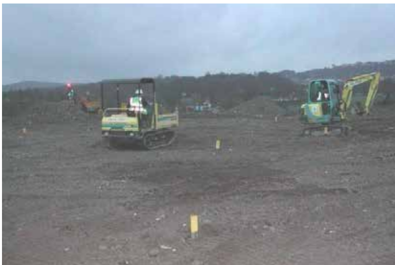
Figure 12: Sludge lagoon at the end of capping operation
