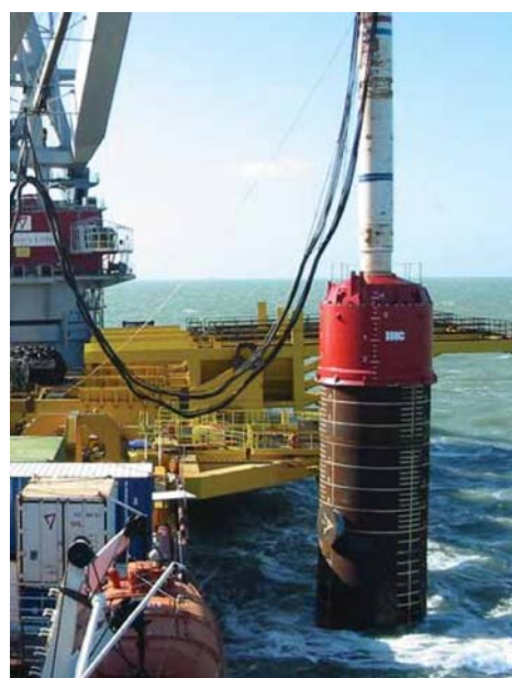
(b) Driving of a 6 m diameter monopile
