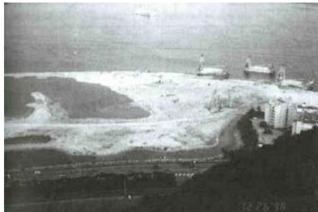
Figure 10: Reclamation works in Pak Shek Kok
