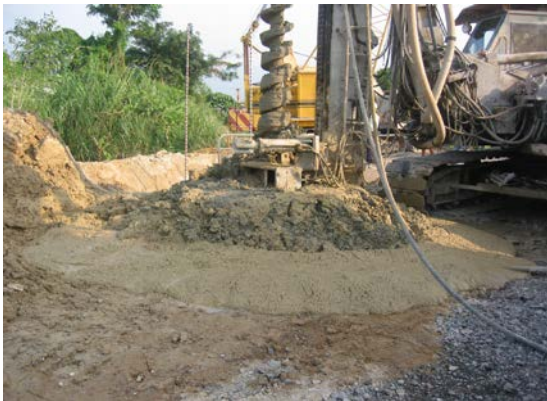
Figure 3: Return slurry deposited at jet grout column A3
