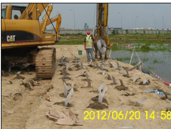
Plate 4: PVD installation in triangular grid
