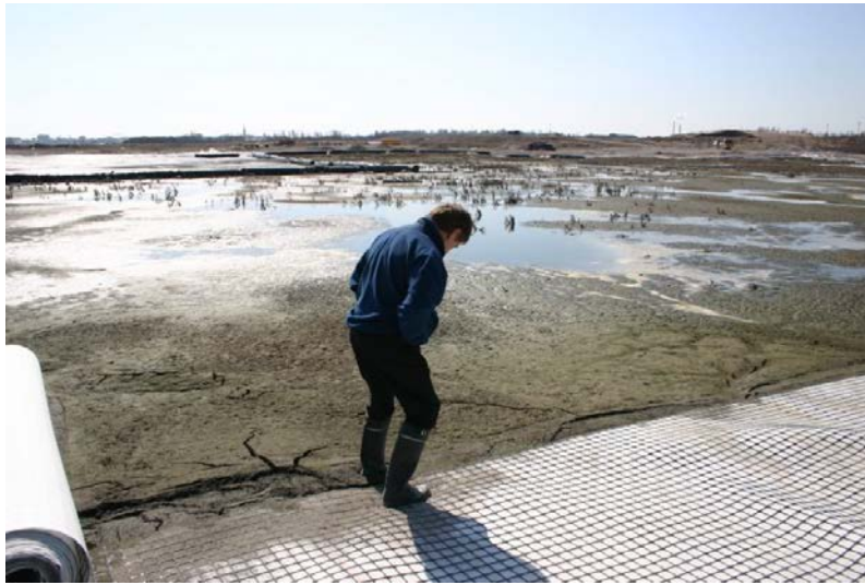
Figure 13: Extremely soft deposits at Heitonen Harbour, Kotka Finland
