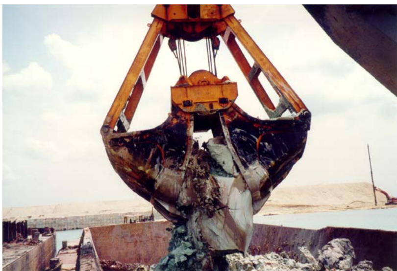
Plate 2: Large stiff clay lump dredged from seabed
