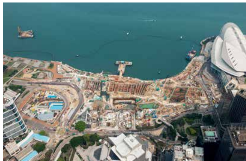
Wan Chai Development Phase II
