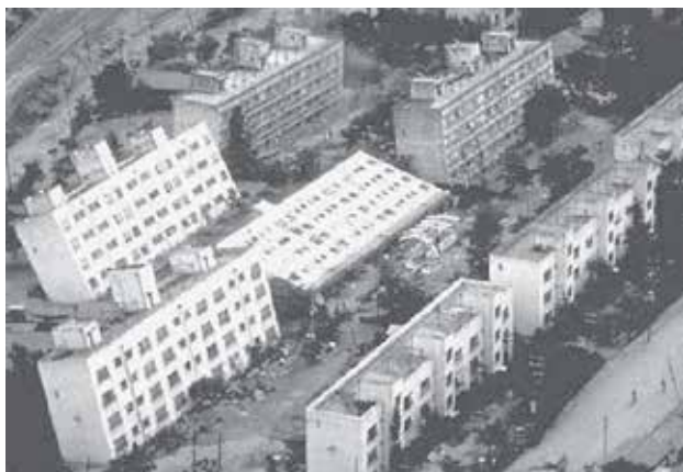
Figure 1: Liquefaction-induced bearing capacity failure of building foundation in the Niigata earthquake in 1964 (Photograph from the Godden Collection, EERC, University of California, Berkeley)
