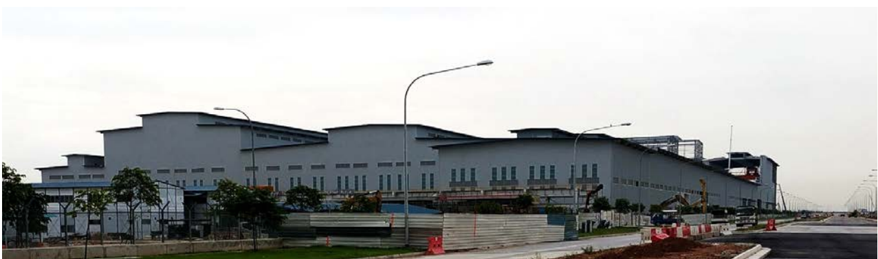
Plate 5: Heavily loaded industrial building built on reclaimed land (photograph taken upon completion)
