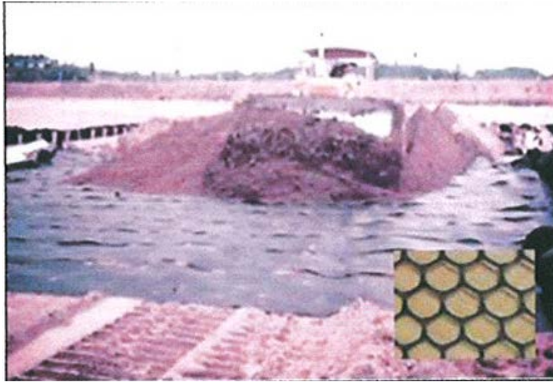
Figure 3: Ground stabilisation on a highway using monolithic geogrids (early 1980's)
