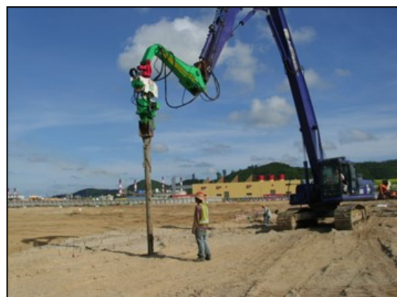
Plate 5: Pre-drilling to facilitate PVD installation
