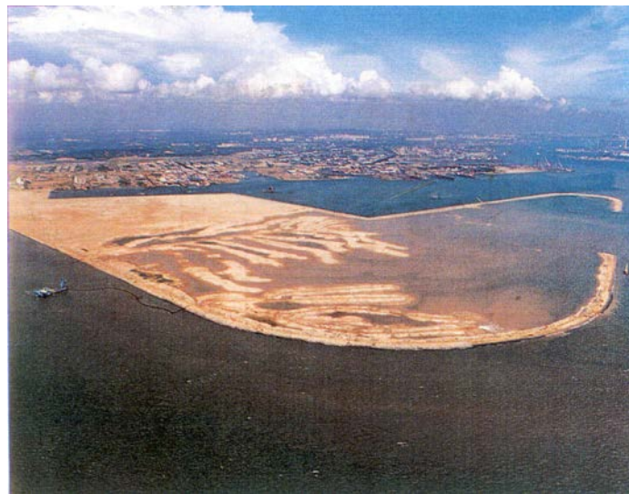
Plate 1: Typical land reclamation work in progress
