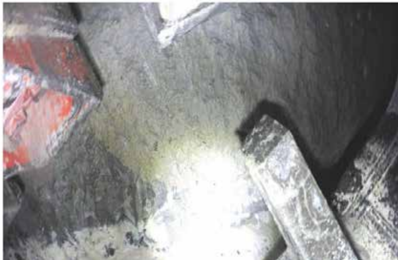
Plate 7: Surface of break-in plug outside TBM cutter head
