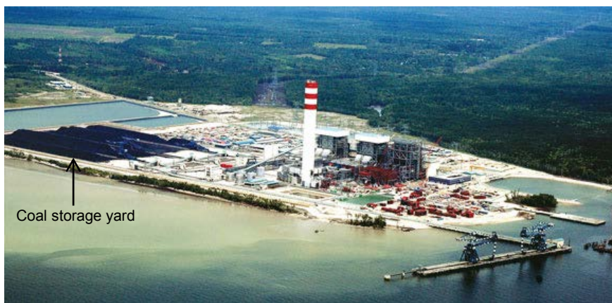
Figure 22: Completed 3x700 MW Power Plant on reclaimed land
