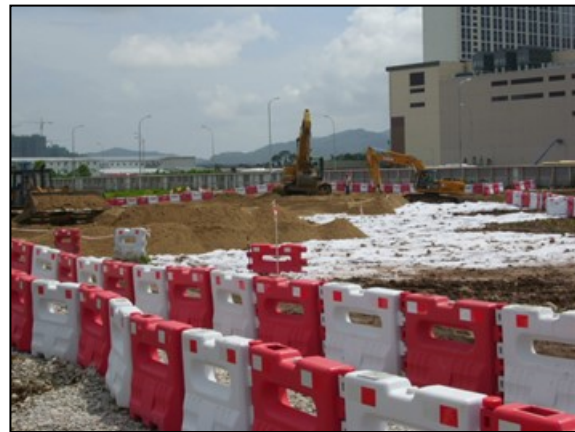
Plate 3: Earthworks separator and drainage layer placement
