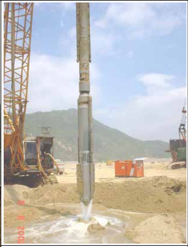
Figure 15: Vibro-compaction
