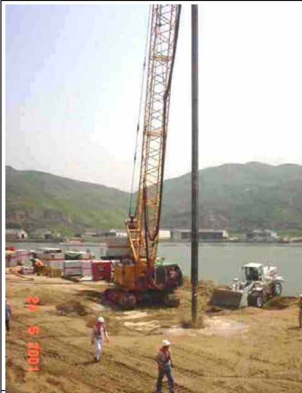
Figure 14: Vibro-compaction
