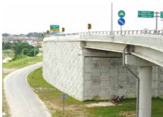
Figure 13: Completed reinforced soil wall, nearly 13 m high.
