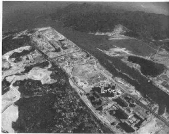
Figure 7: Reclamation works in Shatin
