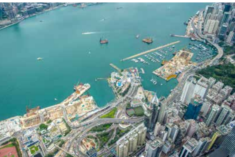
Central - Wan Chai Bypass
