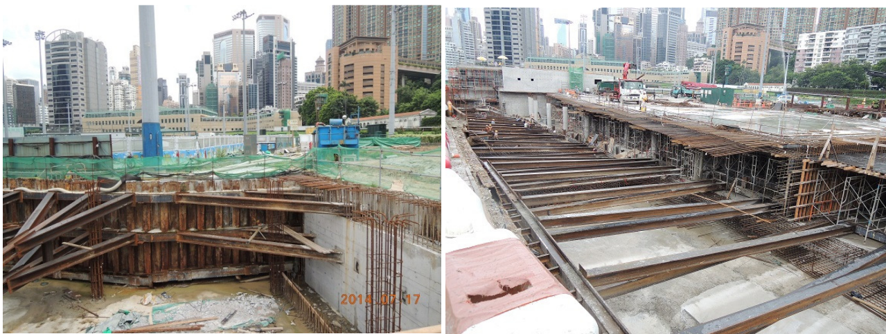
Figure 12: Excavation and Lateral Support Works in Progress
