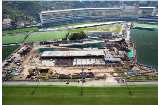
Figure 10: Phase One Construction in Progress May 2014
