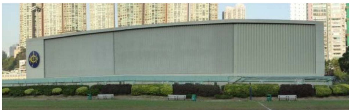
Figure 14: The Diamond Visual Screen on top of LCSD Changing Rooms Building
