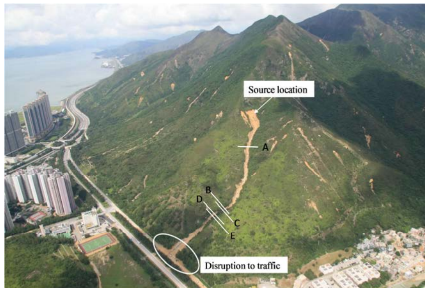
Figure 2: Aerial View of the Debris Flow Event above Yu Tung Road Taken on 9 June 2008
