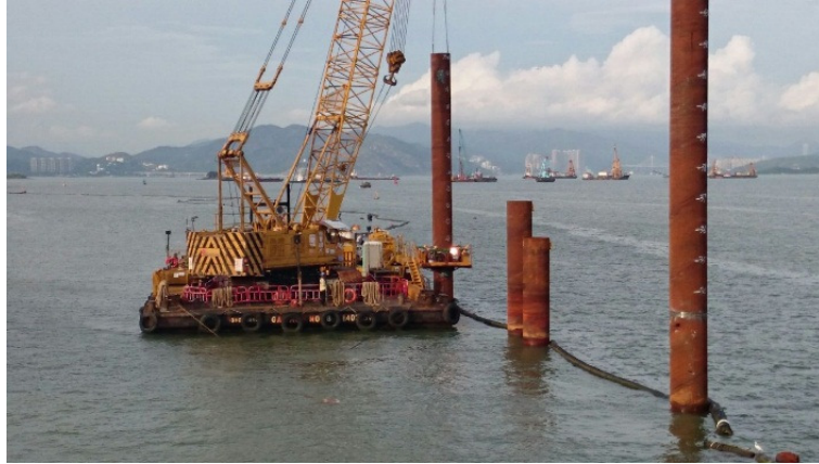
Plate 1: Installation of the Steel Tubular Pile
