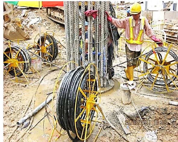
Plate 10: Pressure Grout Injection
