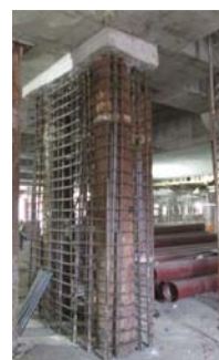
Plate 3 : Steel Fixing for Column
