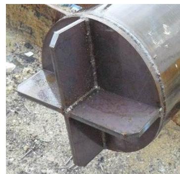
Plate 2: Pile Shoe Detail
