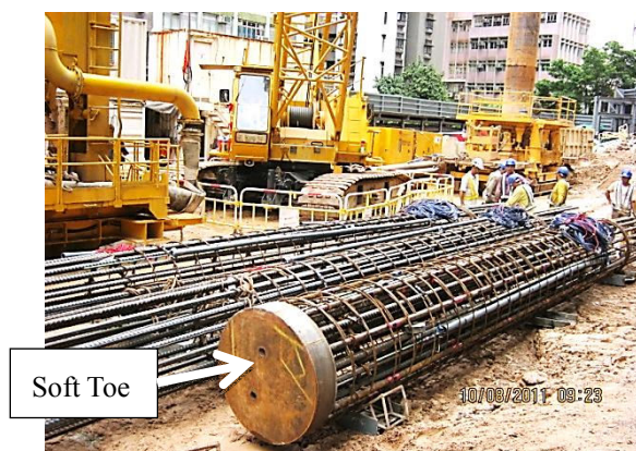
Plate 6: The soft base set up at T-P01
