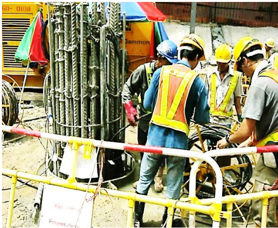
Plate 9: The water cracking process
