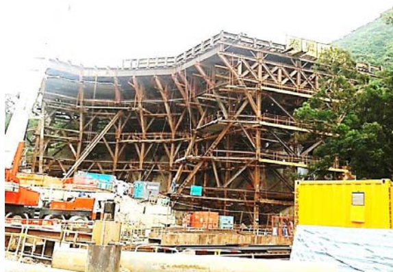
Plate 3: The temporary steel platform for bored pile construction on slope
