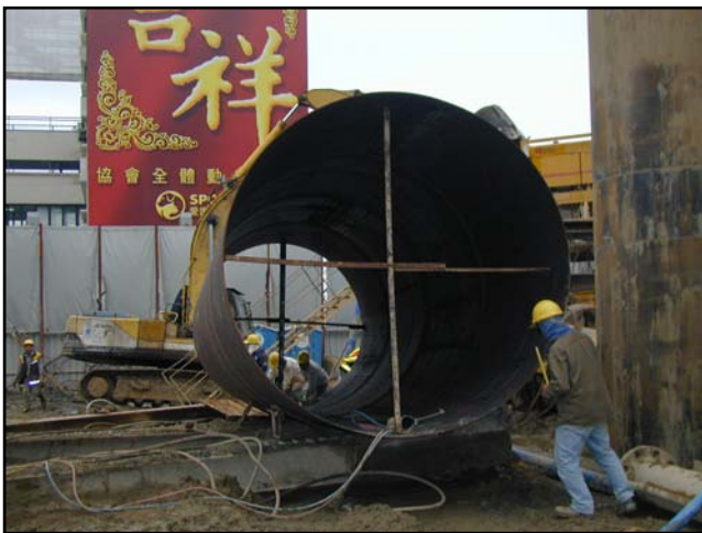
Plate 1: Steel casing for bored pile
