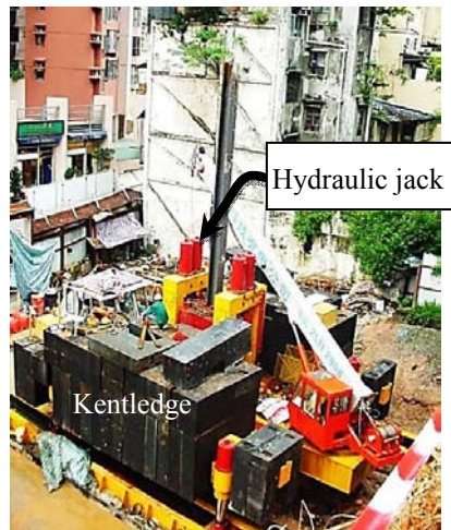
Plate 15: Pile jacking machine at Hollywood Road Site
