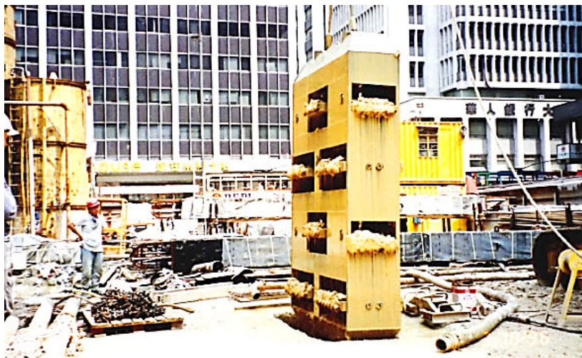
Plate 4: Trench surface scrapping device
