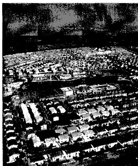
Figure 11: A residential area, Fairview Park in Yuen Long
