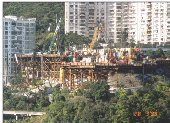
Figure 14 : Similar Gigantic Temporary Working Platform at Stubb's Road
