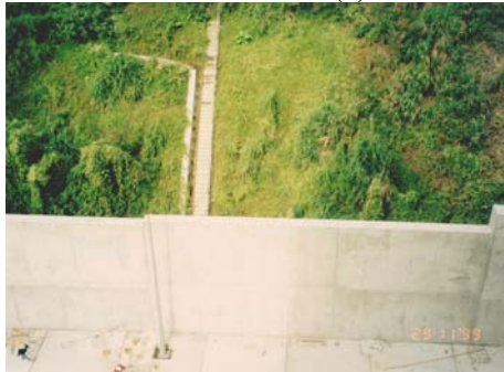
(b) Reinforced Concrete Retaining Wall in Fanling
