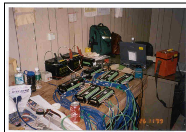
Figure 9 – Central Automatic Data Logging System
