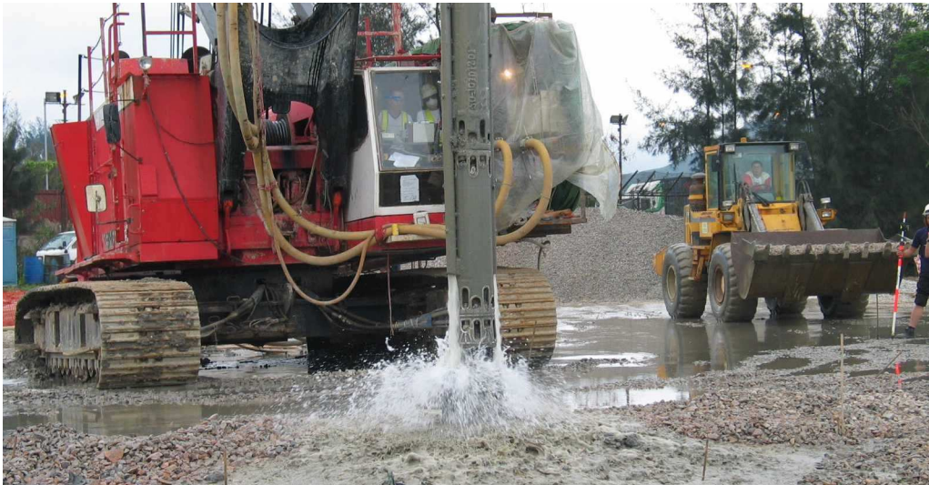
Figure 6 – Installation of Stone Columns by Wet Top-Feeding Process
