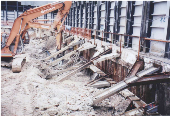
Plate 1 : Existing Basement Trimming Works
