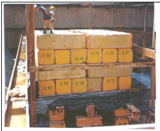
Figure 11A – General View of Plate Load Test Using Conventional Method
