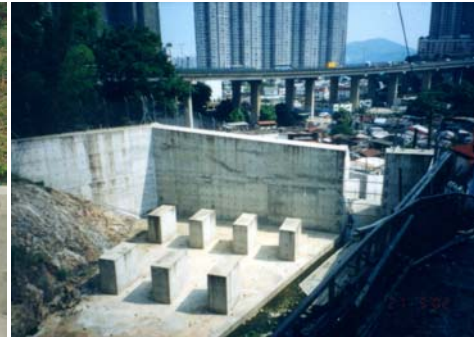
(c) Check Dam in Sham Tseng
