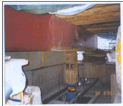
Figure 11B – Testing Set up of Plate Load Test
