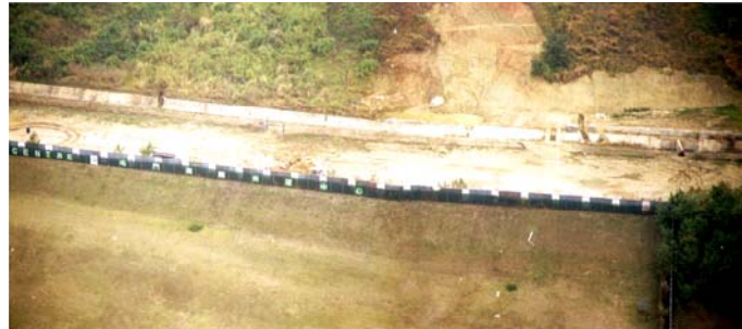
(a) Earthfill Berm in Tuen Mun
