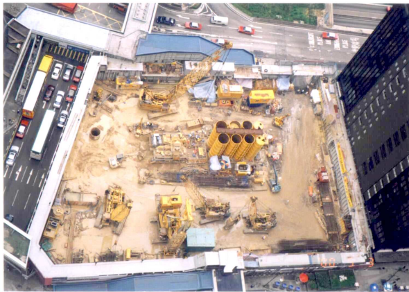
Plate 2 : Aerial View of Foundation Construction
