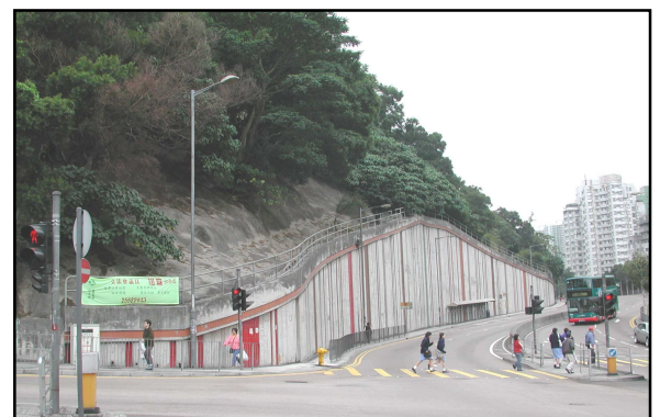
Figure 2 General Appearance of the Wall 15NW-B/CR100
