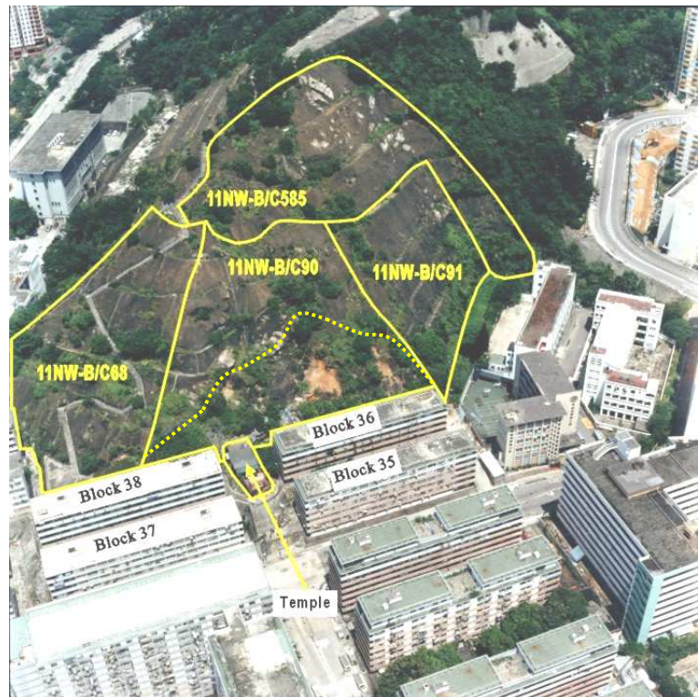
Figure 1 – View of the Slopes (Dotted line shows extent of distressed zone)
