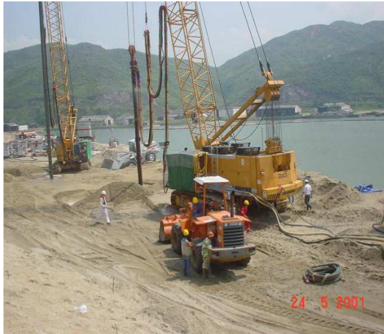
Figure 3 Vibrocompaction in Progress
