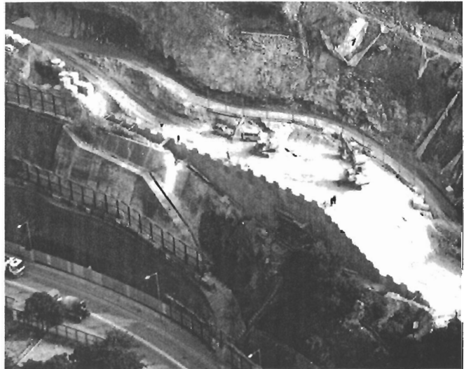
Figure 11 – A 16 m high reinforced fill wall under construction (Lam et al 2001)
