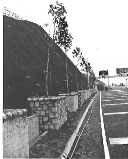
Figure 8 –Establishment of vegetation on a 20m high rock slope
