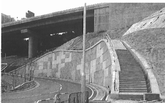
Figure 13 –Architectural finish on a 8m high bored pile wall
