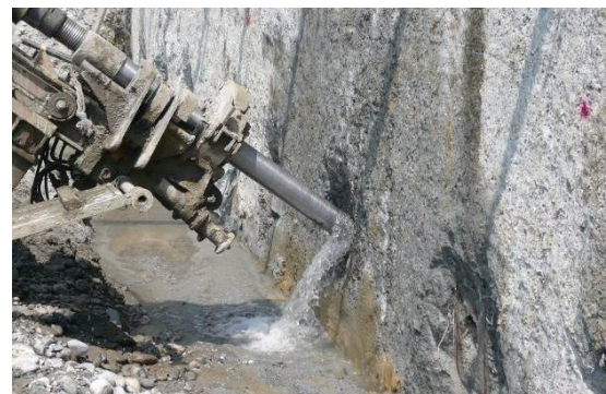
Plate 3: Ingress of groundwater during anchor installation
