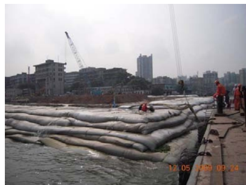
Plate 2: General view of sand bags filled with sand
