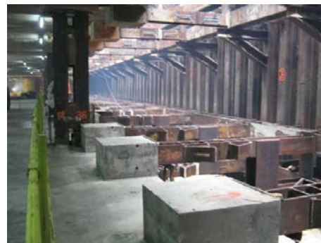
Plate 4: General view of peripheral struts
