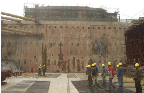
Plate 3: General view of D-wall and anchors
