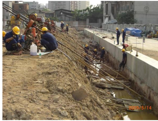
Plate 2: Installation of anchor
