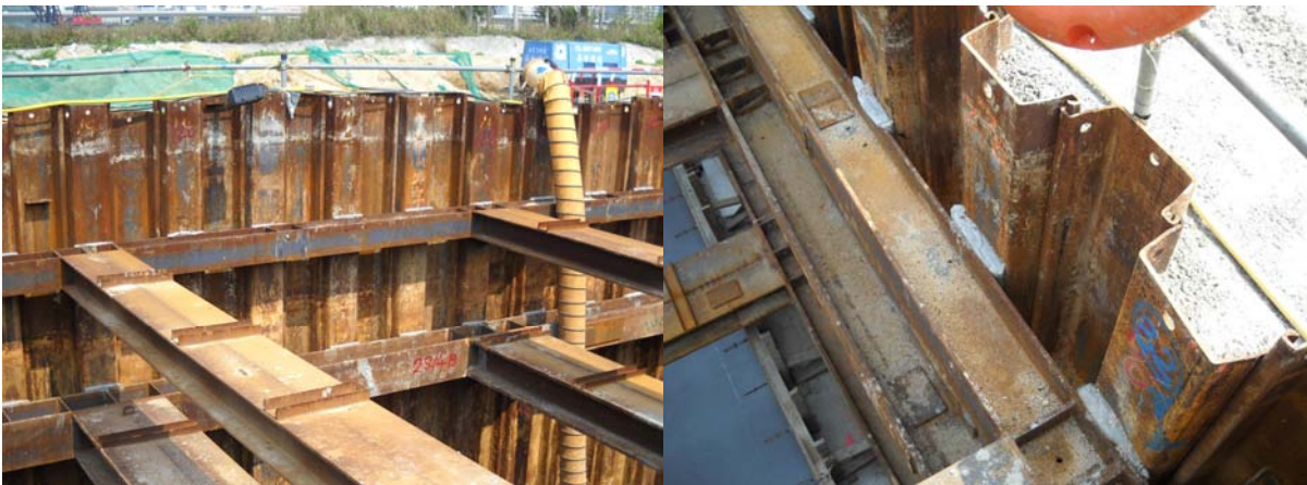
Figure 8: “Double strut” without “splay head”
