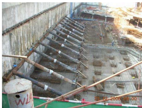
Plate 3: Installed strutting system
