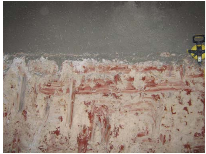
Plate 4: Working shaft exposure, silty clay, uppermost levels
