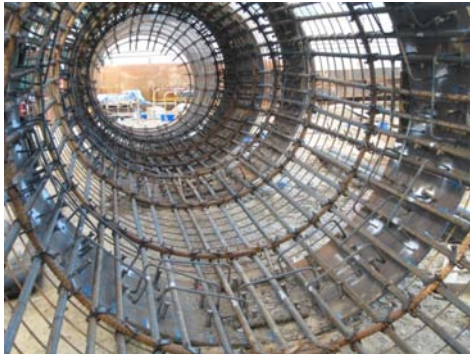
Plate 2: Steel collar in the bored pile
