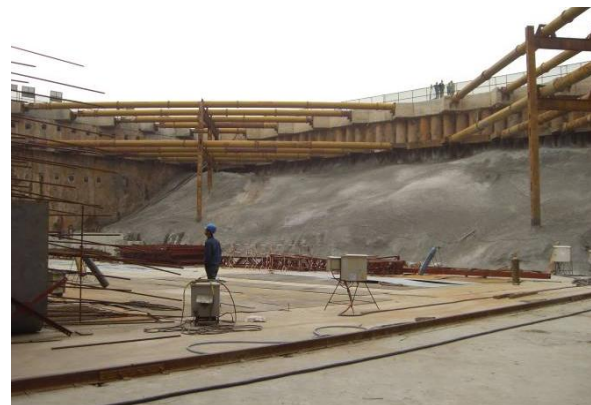
Plate 4: General view of lateral support at river side
