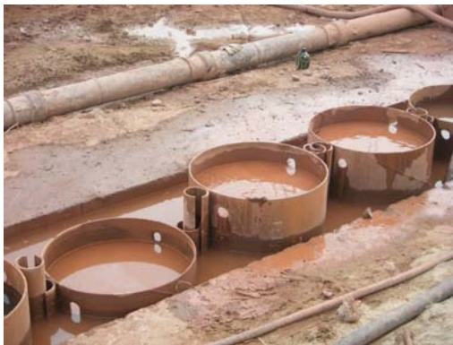
Plate 5: Interlocking of pipe pile wall
