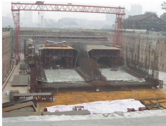
Plate 6: Fabrication of tunnel unit inside dry dock
