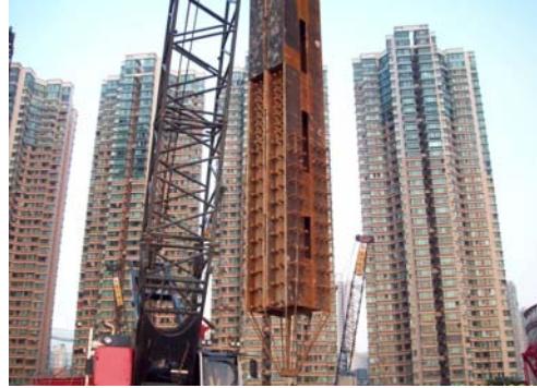
Plate 3: Stanchion installation into bored pile
