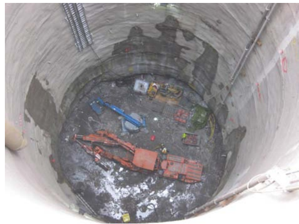
Plate 2: Working shaft excavation
