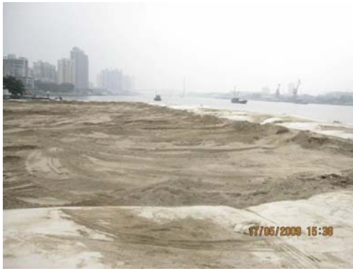
Plate 3: General view of completed reclamation
