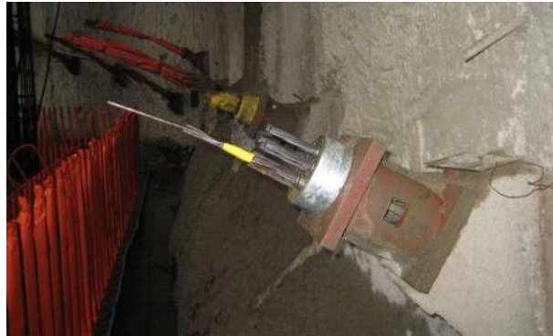
Plate 4: Close-up view of shooting out of individual strands
