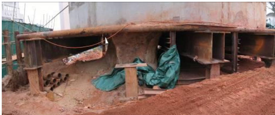
Plate 6: Installation of girder by tunneling method
