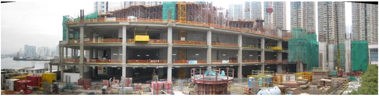
Plate 5: Podium construction concurrently with basement excavation
