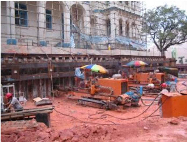
Plate 2: Pilot drill (photo taken from western side)
