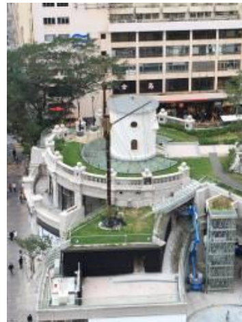
Plate 9: Final preserved signal tower
