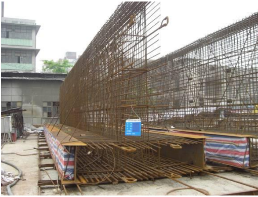
Plate 1: Steel cage fabrication of T-shaped D-wall
