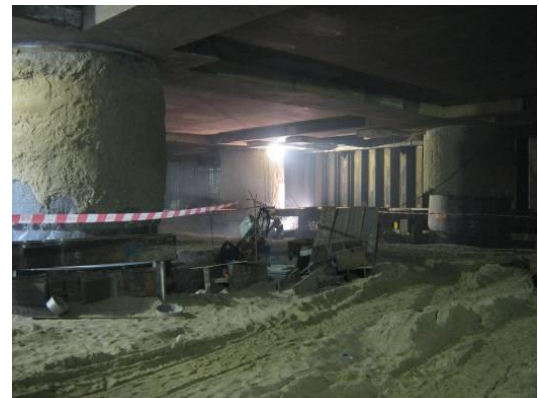
Plate 2: Basement excavation underneath G/F slab
