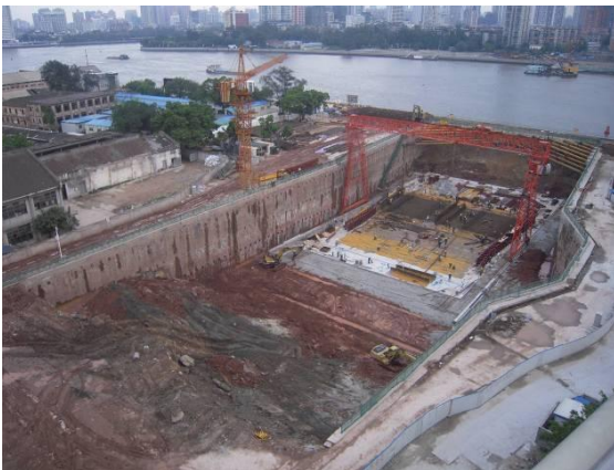
Plate 5: General view of dry dock
