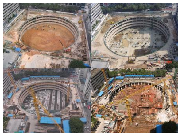
Plate 1: Progress photos for deep excavation and basement construction in Shenzhen
