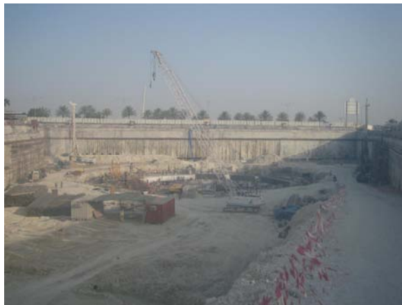
Plate 1: Excavation to level of -12m
