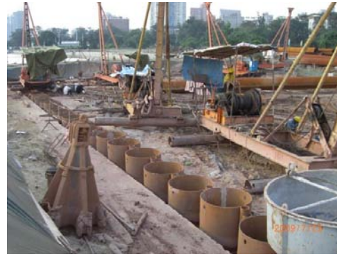
Plate 4: Installation of interlocking pipe pile wall
