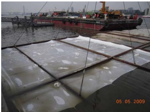
Plate 1: Installation of sand bags for temporary reclamation
