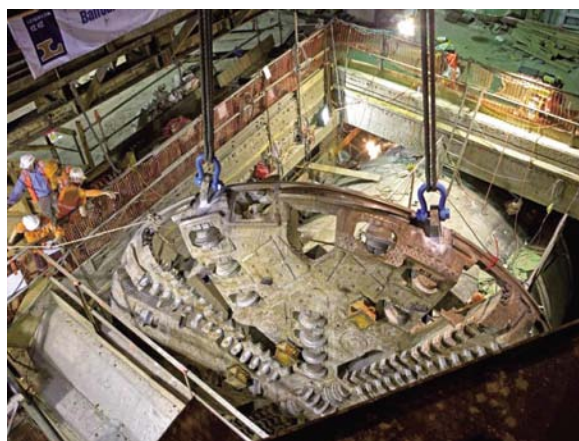
Plate 2: Kowloon Southern Link TBM retrieval.
