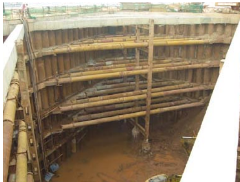
Plate 6: General view of excavation in river
