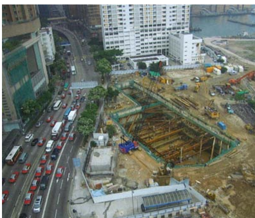
Plate 1: Kowloon Southern Link TBM launch.
