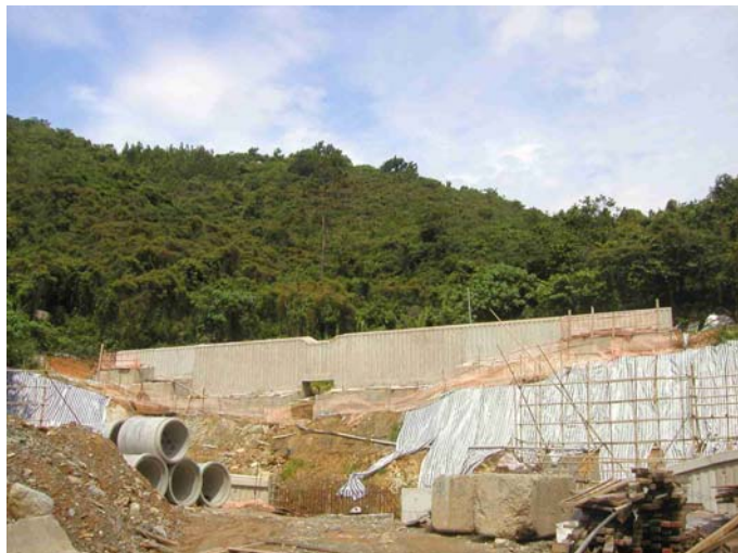
Photo 4: Check dam (Deep Bay Link project)
