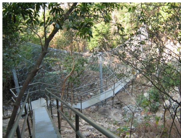
Plate 4: Completed barrier and maintenance accessway
