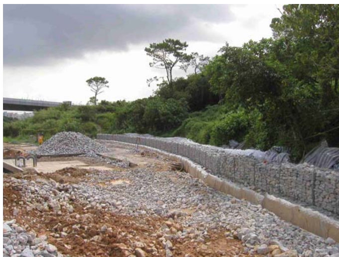
Photo 5: Gabion wall (Deep Bay Link project)
