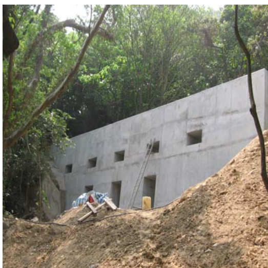
Plate 7: Preventive mitigation measures (concrete check dam with tiebacks concealed in the concrete wing walls)
