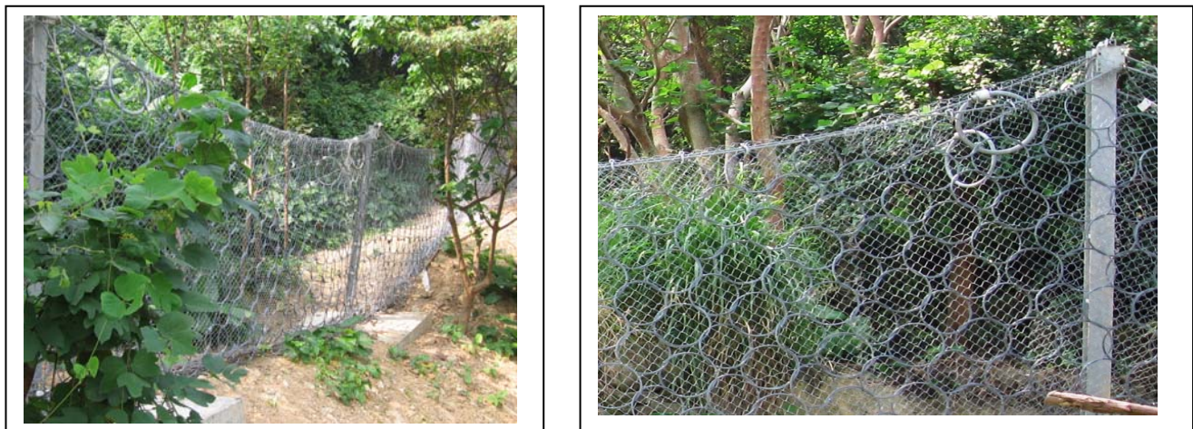
Plate 8: Preventive mitigation measures (flexible barrier with a layer of expanded metal to retain debris)
