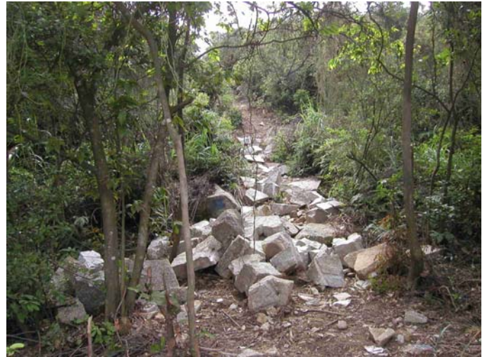
Photo 6: removal of boulders (Deep Bay Link project)
