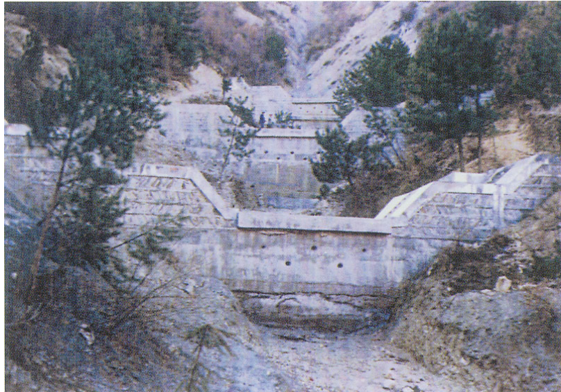
Figure 1: Houshan mountain step-dam is located Heishui county, Sichuan province. These dams with 3-5 m of average high of every step could come into effects in common and protect each other when debris flow hazards occur
