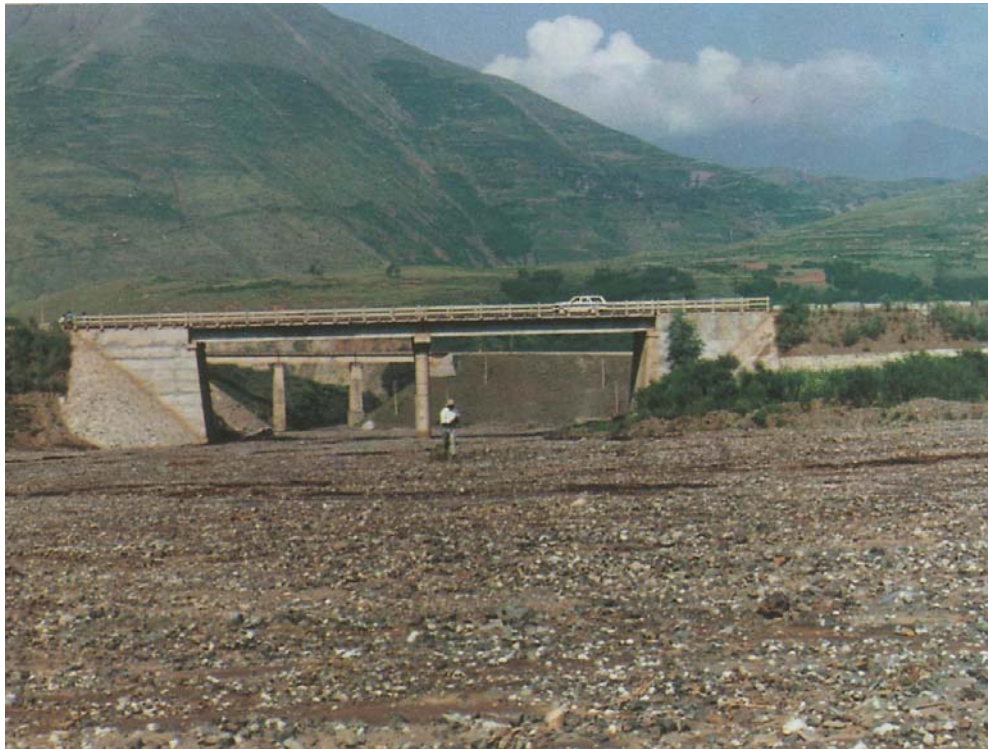
Figure 6: Xiaohaihe Road and Railway Bridge is located in Dongchuan city, Yunnan province and keeps road and railway running in security because the turbulent debris flow and mountain torrent could pass through it in safety
