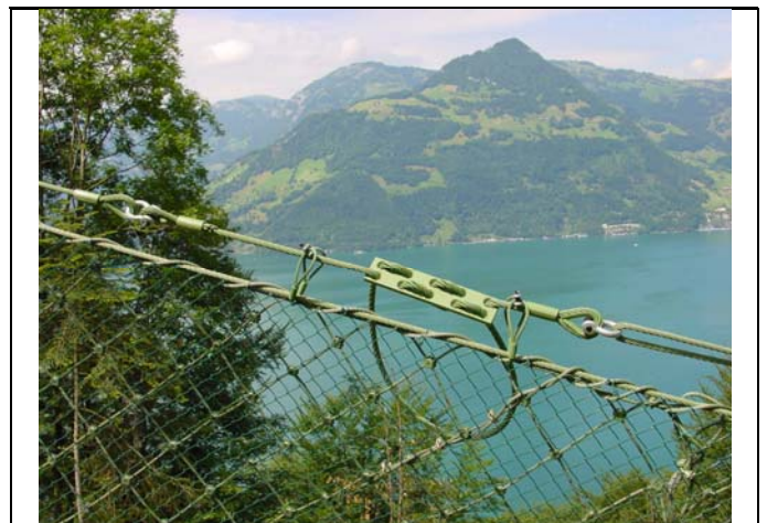
Plate 2: Specially-designed rope brakes
