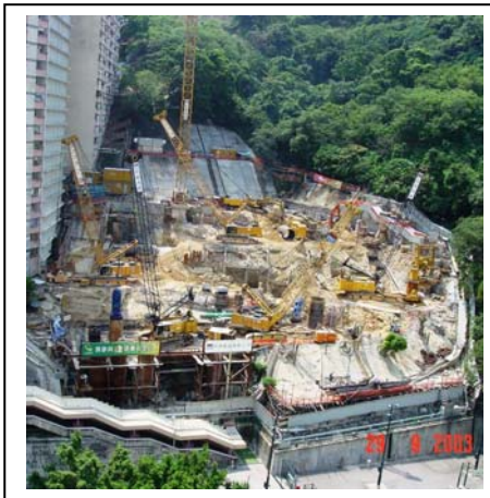
Plate 2: Site formation works at toe
