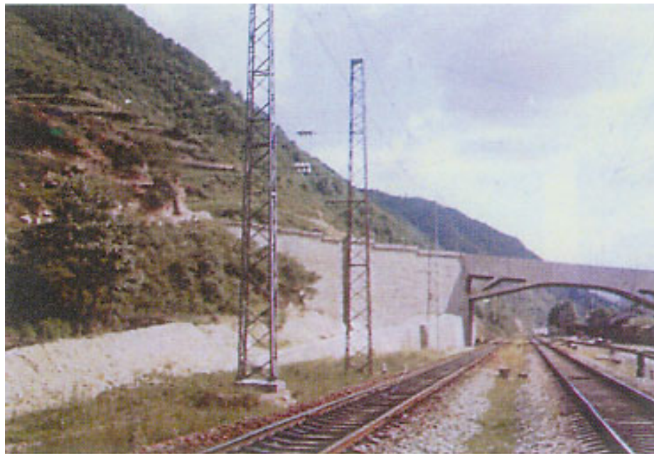
Figure 7: The road or railway could pass through in the lower of eroded line of debris flow when the protection entity is lower than debris flow. Debris flow could reach the lower of debris flow valley through drainage slot. This is a debris flow drainage slot across Baoji-Chengdu railway in Feng county, Shaanxi province
