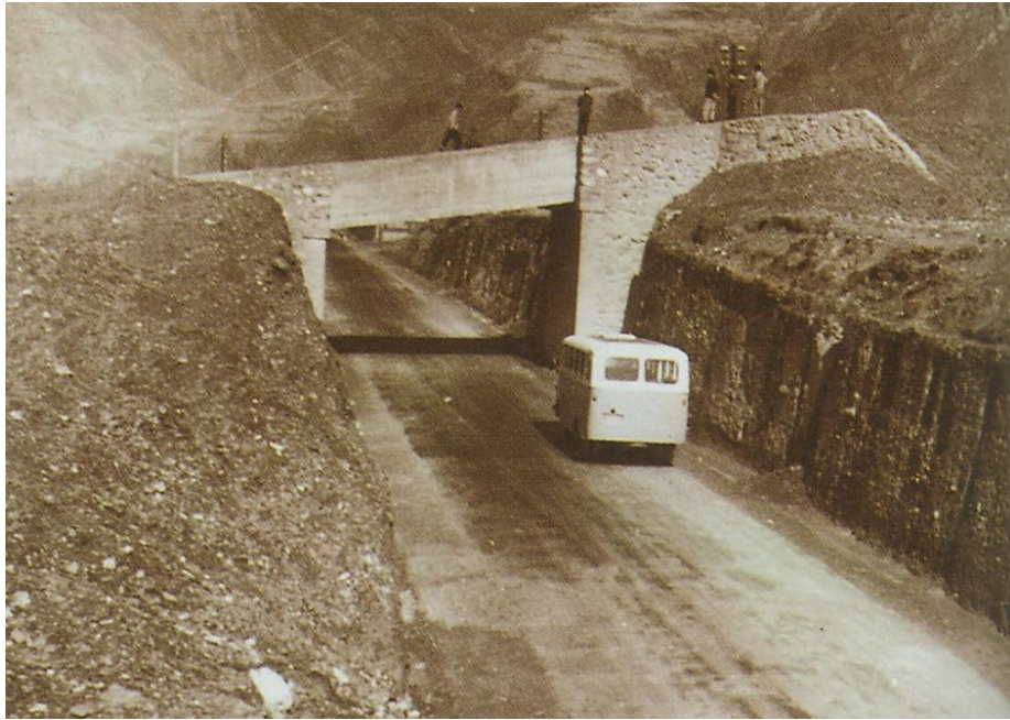
Figure 8: The Drainage slot across debris flow valley in Wudu county, Gansu province
