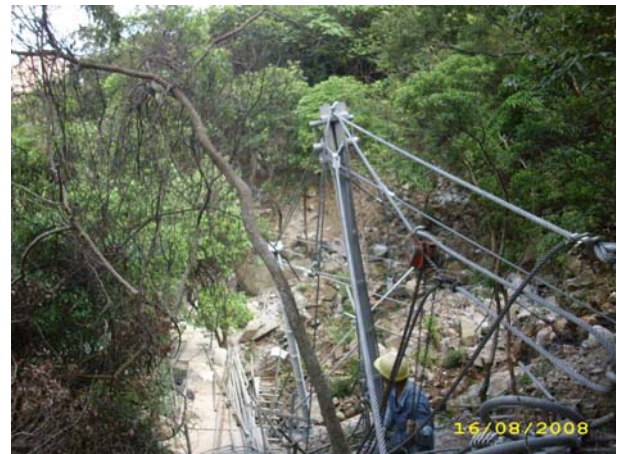
Plate 1: Erecting hinged post
