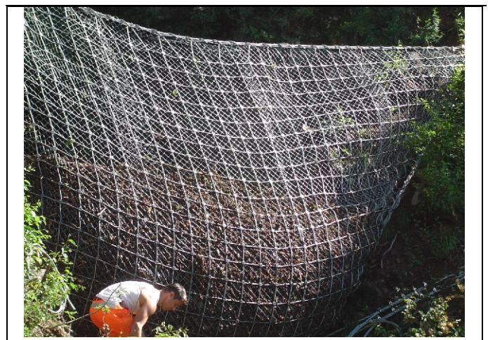
Plate 1: Diagonal net with clamp
