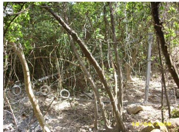
Plate 2: Fixing brake rings
