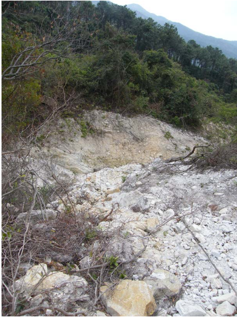
Plate 3: Disaggregated colluvium in the foreground is located in the middle part of the slide. Distal debris below the far trees are remnants of the landslide toe on the far side of the debris flow channel. The remainder of the landslide toe has been removed by post-landslide erosion
