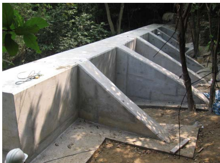
Plate 7: Preventive mitigation measures (concrete check dam with tiebacks concealed in the concrete wing walls)
