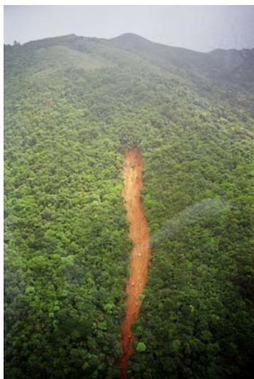
Plate 1: Oblique aerial view of the August 2005 landslide
