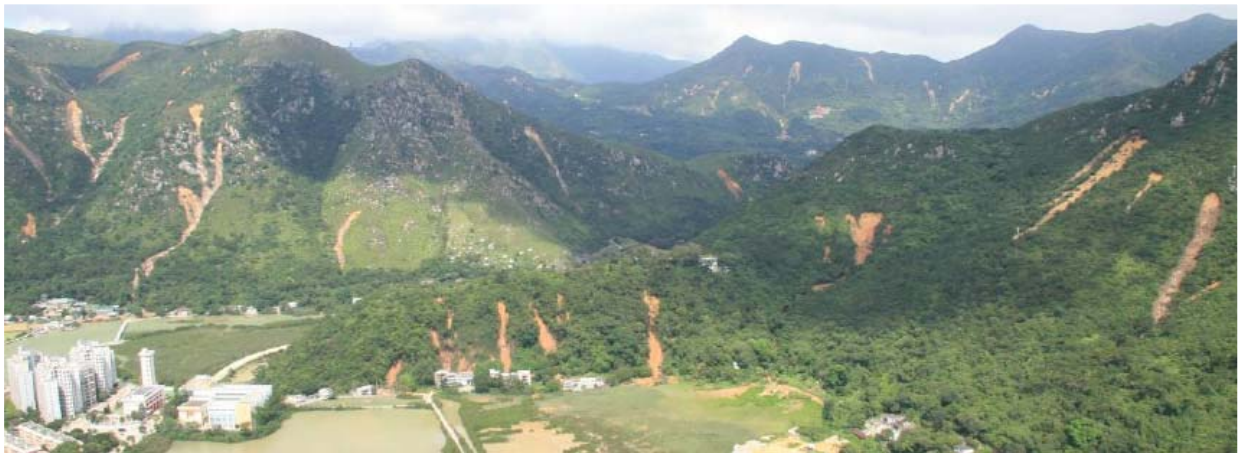
Figure 10: Landslides in Tai O, Lantau in the June 2008 rainstorm
