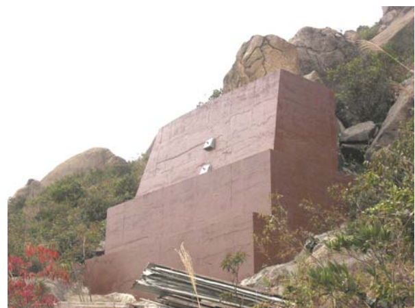
Photo 2: Buttress (Nam Wan project)
