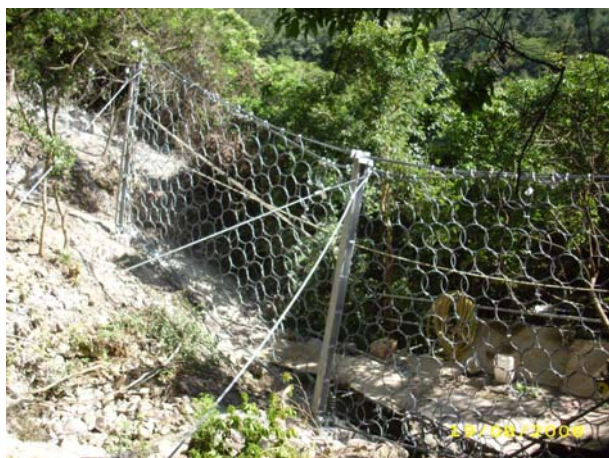
Plate 3: Mounting ring net
