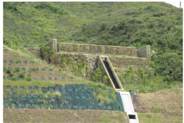
Plate 4: General layout of DBR after landscaping works
