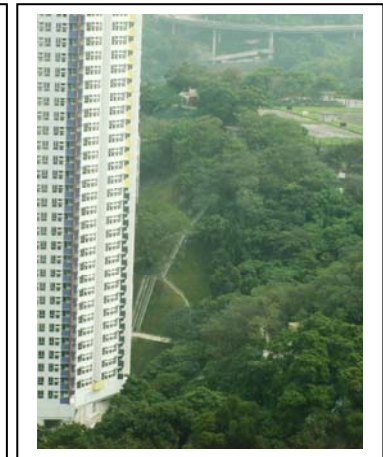
Plate 3: Completed building at toe
