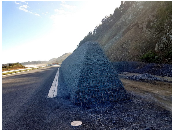
Figure 6: Earth bunds for slope production in Kaikoura.
