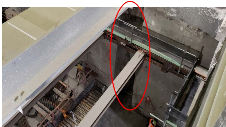
Figure 22: Jet grout column between Diaphragm Wall panels.
