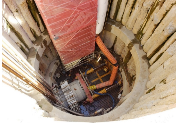
Figure 4: Pipe-jacking TBM launching shaft for City Rail Link Contract 6.
