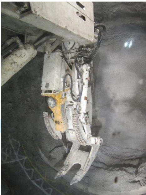
(a) Manipulating demolition arm for segment dismantling
