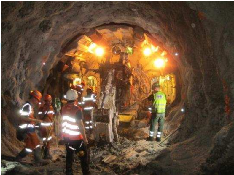
Figure 21 Demolition chamber during an atmospheric stop
