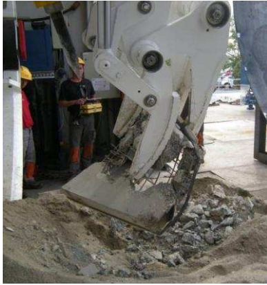
(a) Breaking of segment by hydraulic breaker
