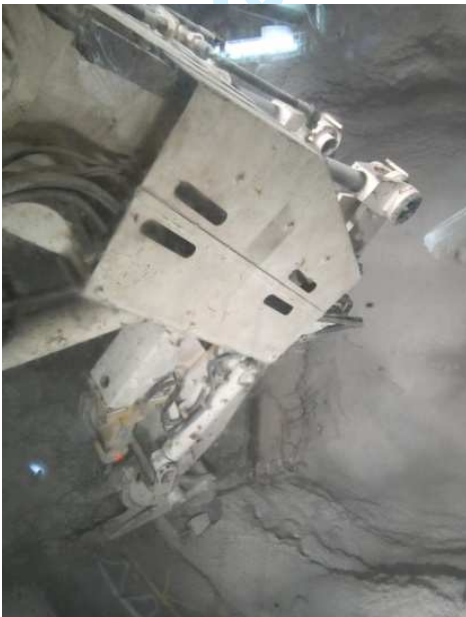
(b) Shotcreting operation
