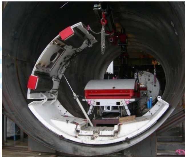
28 (a) Testing of hinged joint in mock-up tunnel
