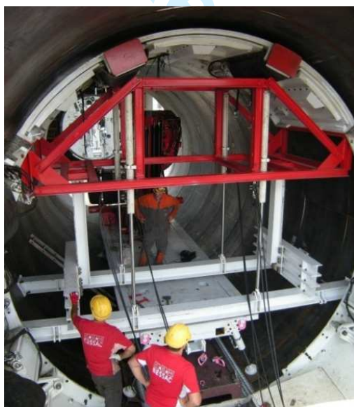
50 (b) Testing of jacking frame in mock-up tunnel
