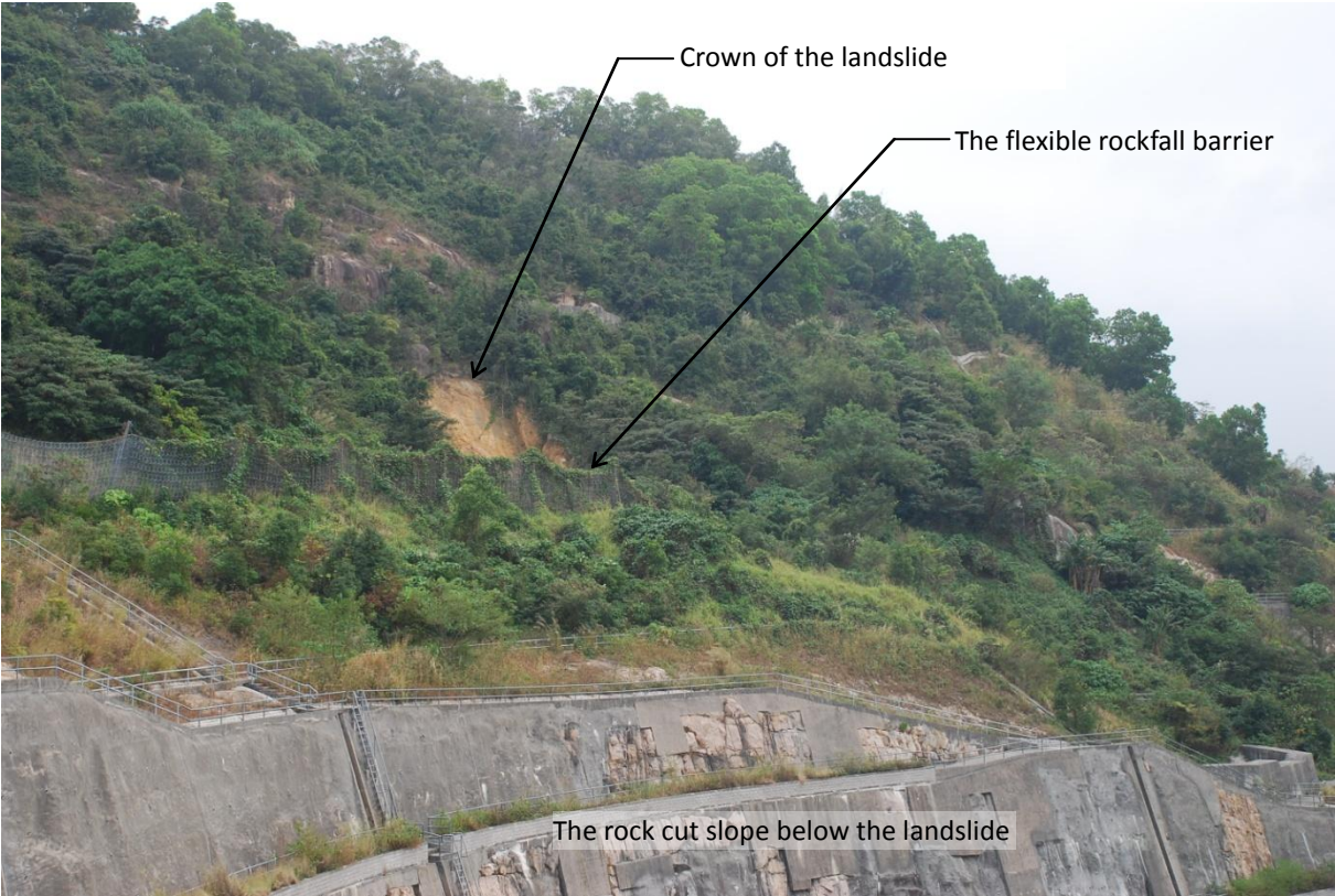
Figure 1 An overall view of the landslide site
