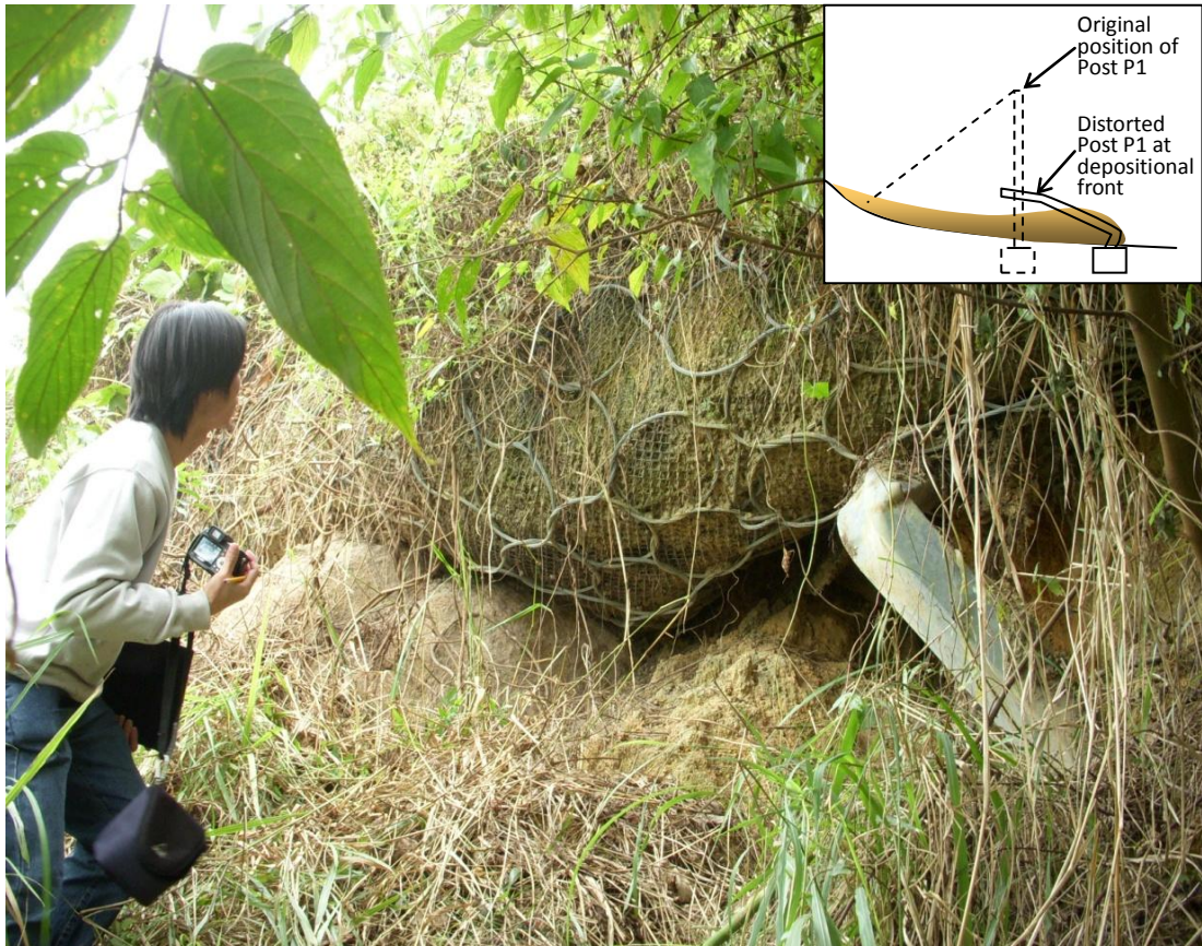
Figure 5 Post P1 damaged; landslide debris was largely contained by the barrier
