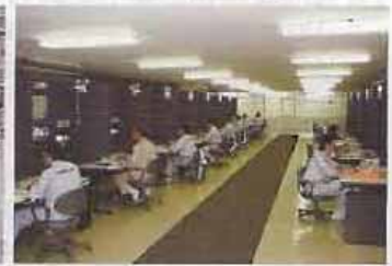
Picture.2 Ground remote control cabin in unmanned excavation
