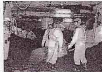
Picture.5 Personnel servicing excavation equipment in the working chamber
