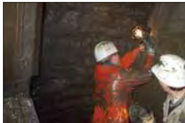
Regular inspections in cutter head
