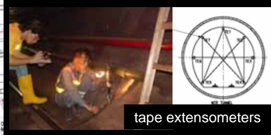
84 strain gauges + seismographs
