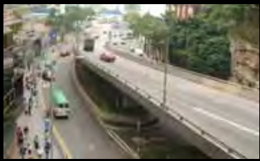
view of bridge structure
