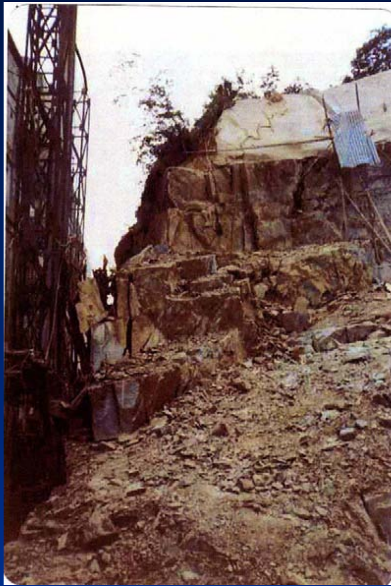
Eastern part of slope before failure
