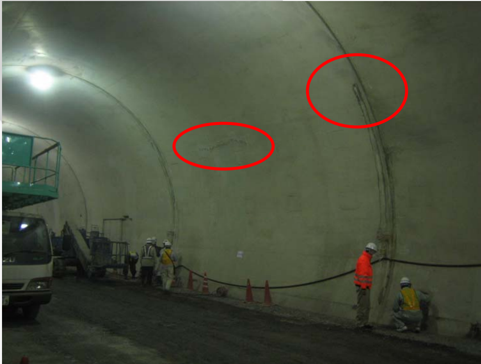
Final Tunnel shell with wet areas
