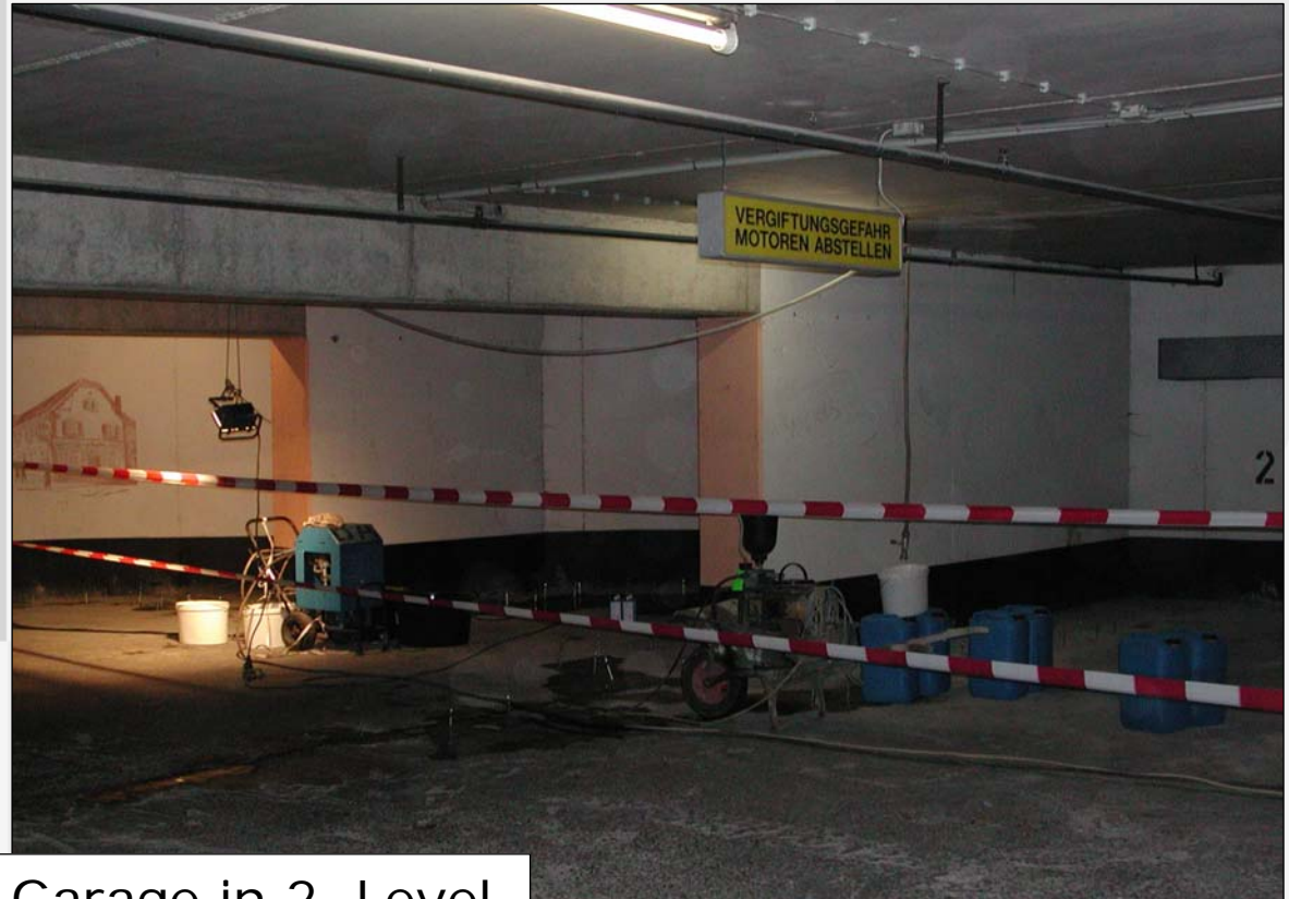
Site overview: Parking Garage in 2. Level
