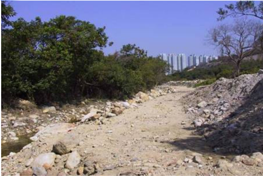
Tung Chung River - before reinstatement
