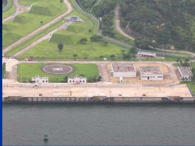
KSW Explosives Depot
