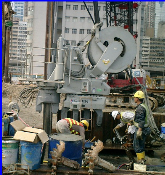
Sheetpiling by push-in method
