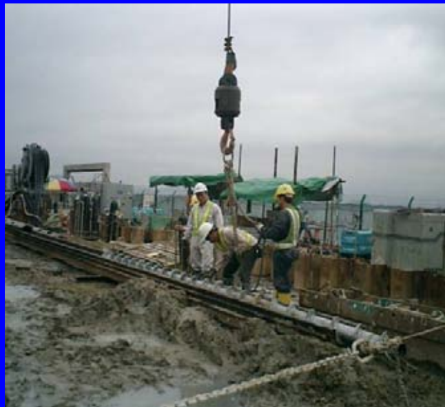
Augering to assist penetration
