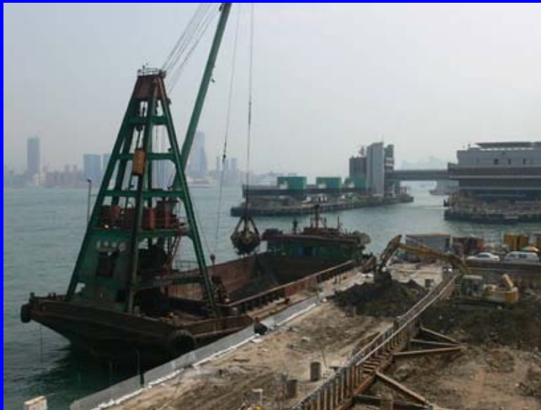
Disposal by barge
