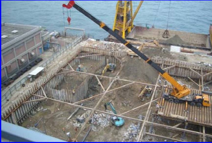
Excavation in progress
