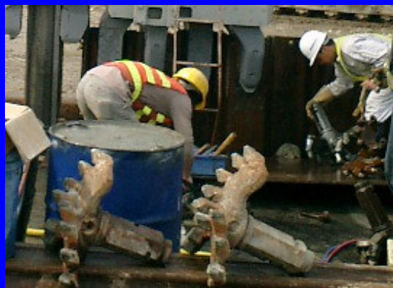
Cutter Head for Rock Obstructions
