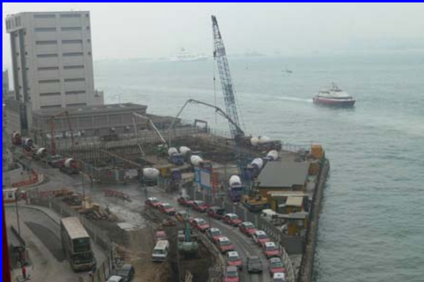
Concreting in progress (3 concrete pumps & 13 concrete trucks)
