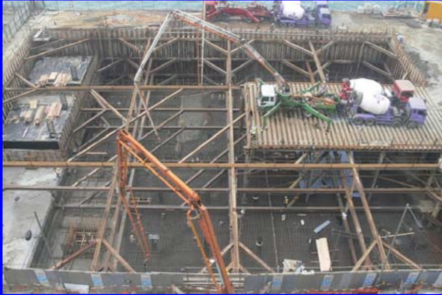
Concreting in progress
