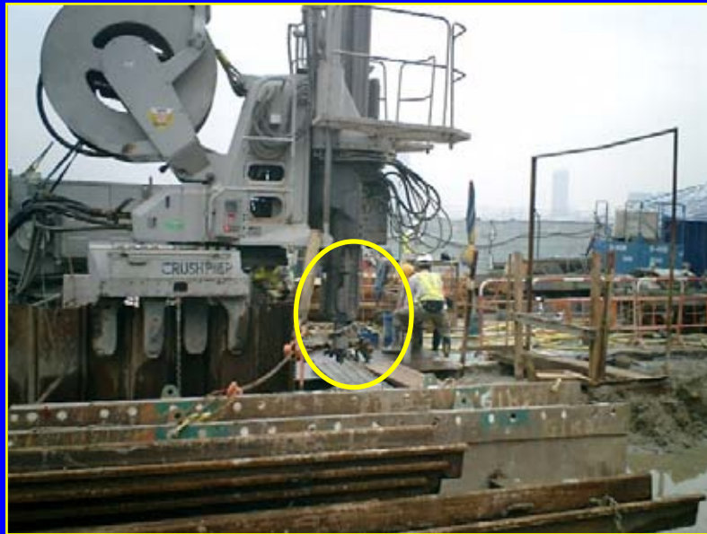
Drilling through Obstructions
