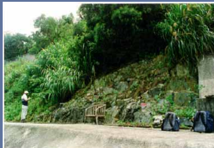
Plate 3 - General View of Planar, Obliquely Outward-dipping PW0/30 and PW90/100 Rock Mass Weathering Zone Interface (84356 81362), Associated with Kaolinitic Clay Development, in Slope 11SE-D/C188, West of Siu Sai Wan Estate (Taken 17/7/96)
