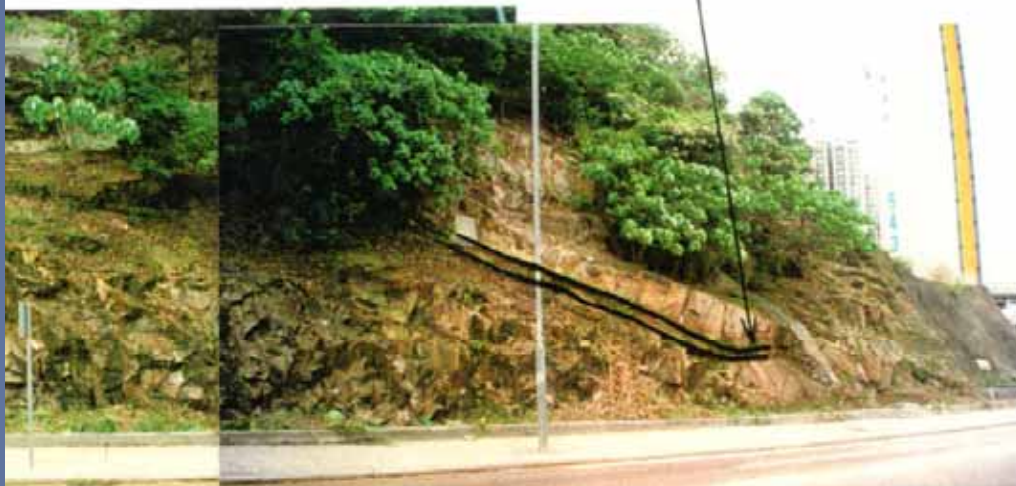
Plate 3 - General View of Planar, Obliquely Outward-dipping PW0/30 and PW90/100 Rock Mass Weathering Zone Interface (84356 81362), Associated with Kaolinitic Clay Development, in Slope 11SE-D/C188, West of Siu Sai Wan Estate (Taken 17/7/96)
