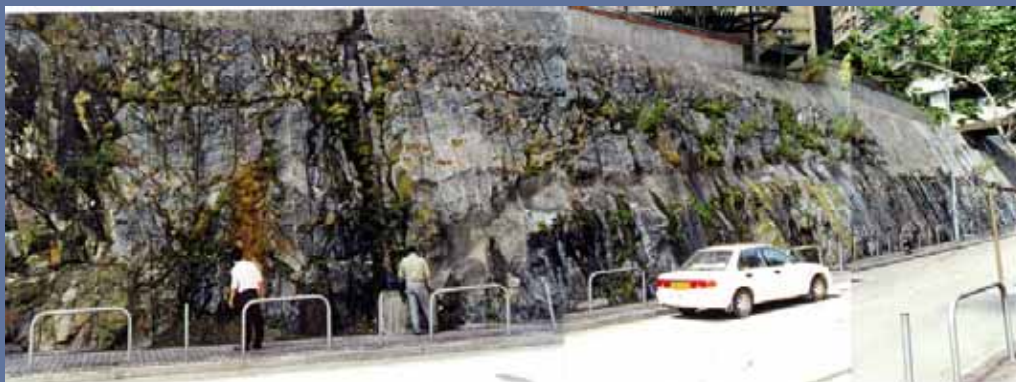
Plate 6 - Unregistered Slope 15NW-3B/S10 (834250E 811530N), in Lei Tung Estate Showing a Relatively Planar Weathered Seam (Largely Covered by Chunnam) of Kaolinitic Clay, c.150 mm Thick, Dipping c.30-35° out of the Slope at about Mid-height within Grade II Tuff. Extensive Groundwater Seepage was Noted from the Seam during Site Inspection. (Taken 12/11/96)
