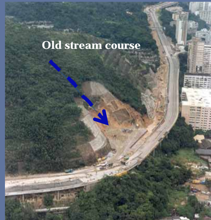
Ching Cheung Road Landslide in 1997
