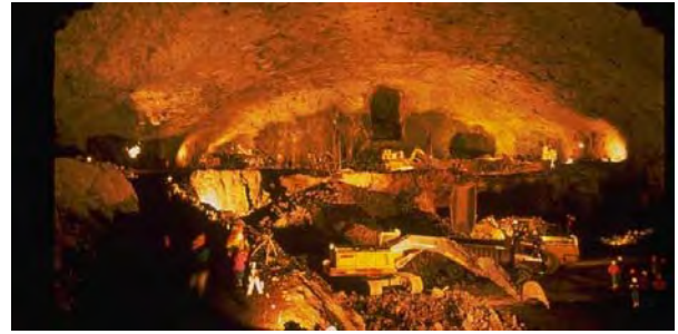
Fig. 3 Excavation Sequence Gjøvik Hall (Photo: NGI)
