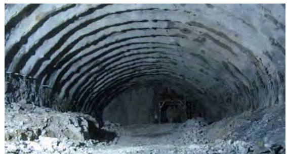
Fig. 5 Ribs of Shotcrete Reinforced with Lattice Girders in a Large Underground Hydropower Cavern
