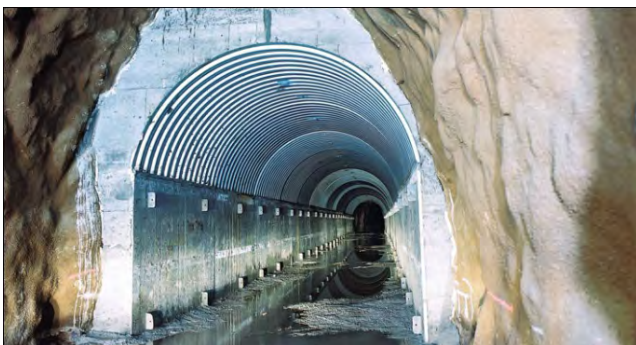
Fig. 11 Tunnel from Lake Päijänne was Repaired the First Time in 1999 (Photo: Photo Mannelin)
