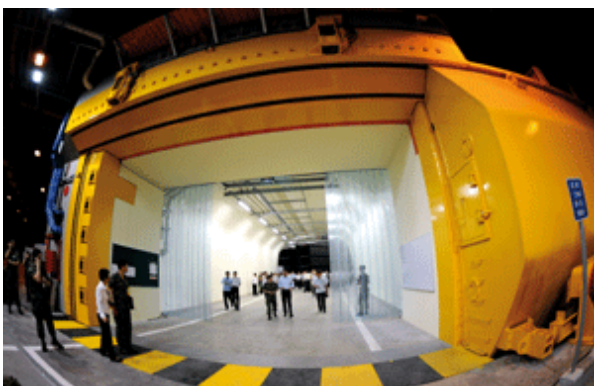
Fig. 2 Singapore Ammunition Storage
