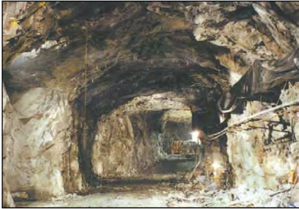
Fig. 6 Record Photo of Cavern Excavation
