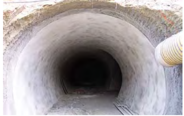
Fig. 2 Wine Cave Entrance after Application of Spray-on Waterproofing Membrane
