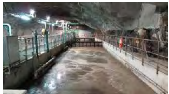
Fig. 4 Overview of the Aeration Tank
