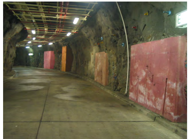
Fig. 3 Rock Buttresses Installed in the Tunnel
