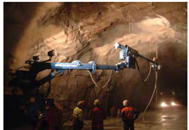
Fig. 3 Spraying of Intersection with Computer Controlled Equipment – Nordøy Tunnel
