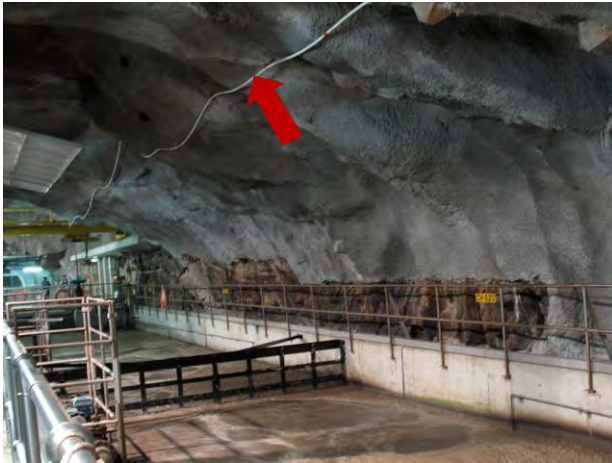
Fig. 9 Typical Example of Smoke Detection System
