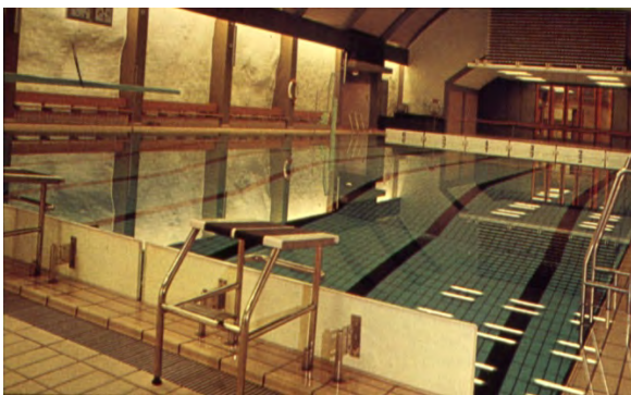
Fig. 9 Combined Underground Sports Facility and Civil Defence Shelter (Photo unknown)
