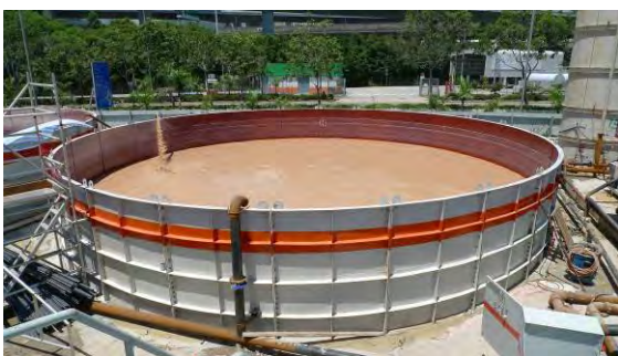
Fig. 11 Steel Circular Bentonite Pool, 400 m 3 Capacity
