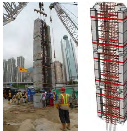
Fig. 13 Installation of Rebar Cage with SVF
