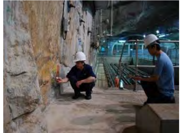
Fig. 12 Conduction of Geotechnical Survey
