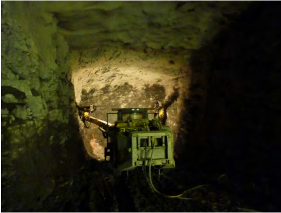
Fig. 7 Excavation of the Center Drift of the Top Heading
