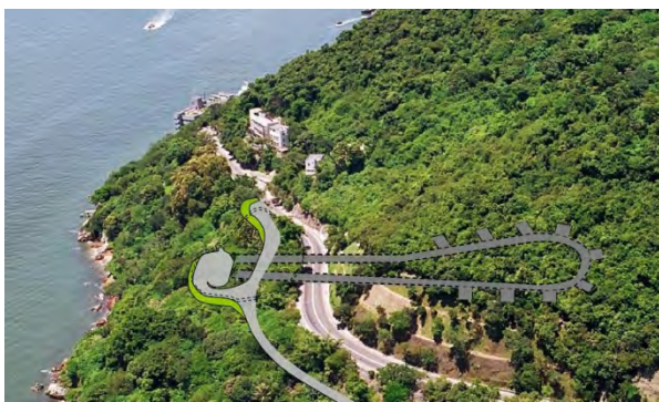
Fig. 6 Oblique Aerial View of Underground Magazine Site South of Victoria Road
