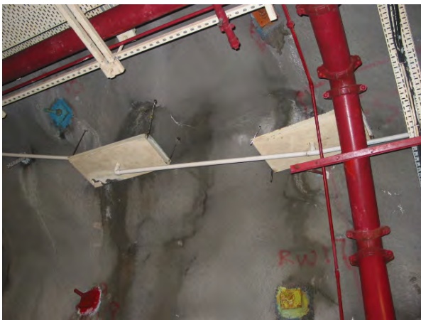
Fig. 4 Waterproofing Works (Drip Trays) Installed to Protect Pipelines in the Tunnel
