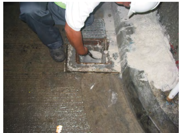
Fig. 5 Removal of Lime Accumulation from the Subsurface Drains in the Tunnel
