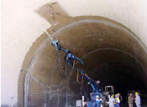
Fig. 4 Computer Controlled Spraying – Chekka Tunnel
