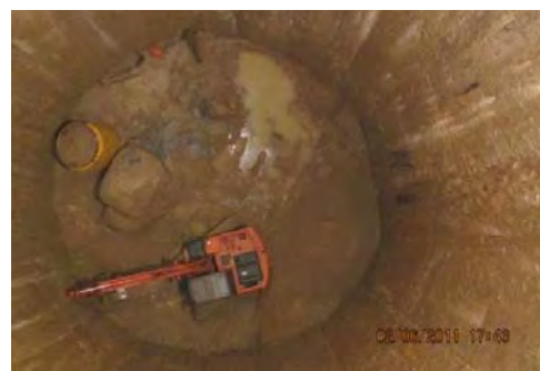
Fig. 14 A 13 m Dia. Shaft under Excavation at 82 m Depth (with the application of SVF, diaphragm walls are in perfect alignment)
