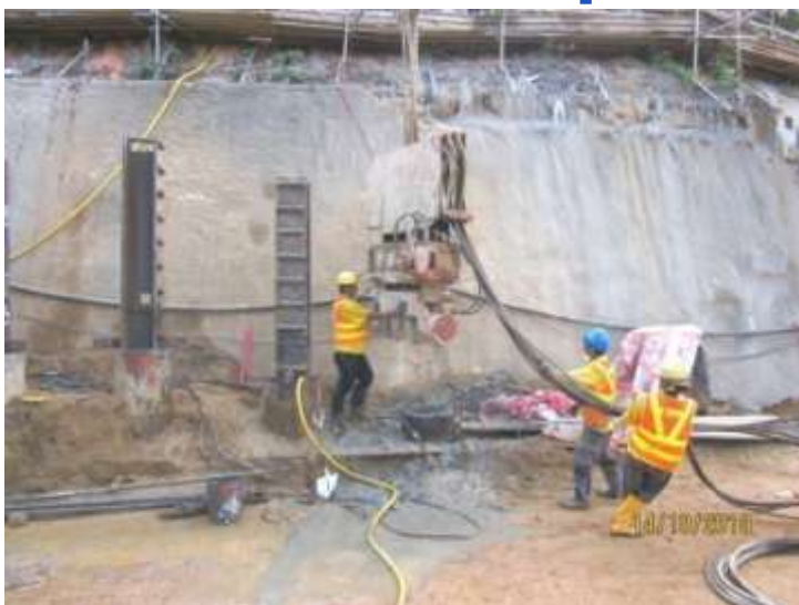
4. Extracting Temporary Casing
