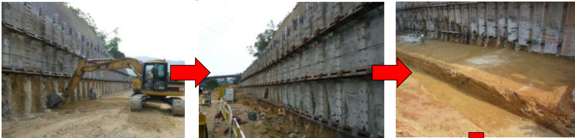
8. Excavation down to Formation Level of Stabilizing Base
