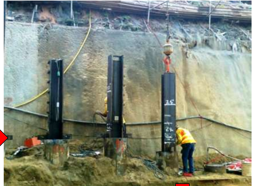
2. Inserting H-pile
