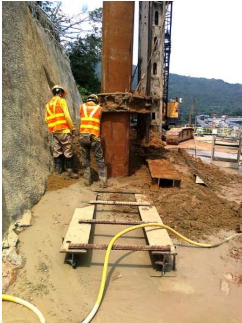
1. Pre-boring with guard-rail
