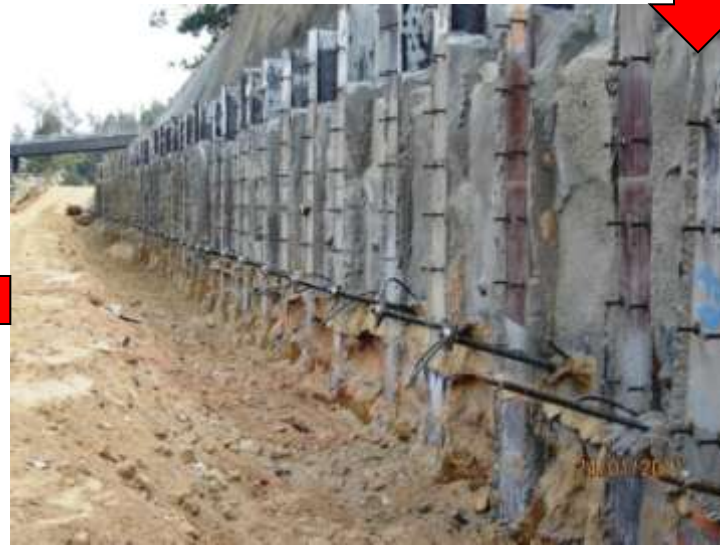
6. Installation of shear stud & Temporary Tie-back
