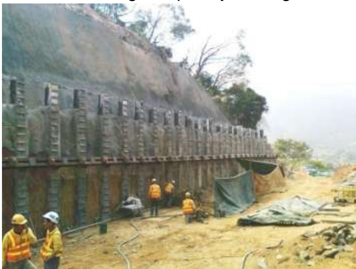
7. Installation of waling
