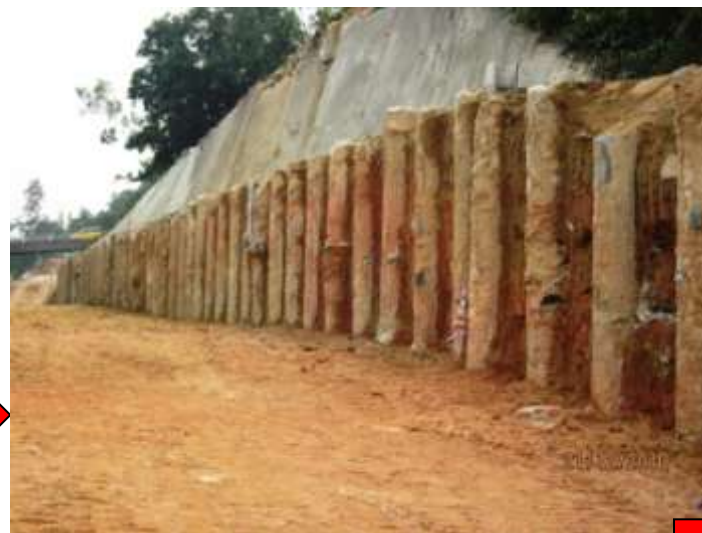
5. Excavation in front of Soldier Pile
