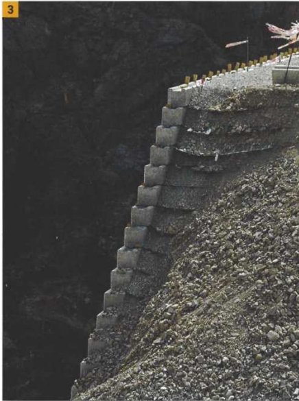
1. Construction of the 20m high earth-retaining reinforced walls 2. A cut section through the rugged mountain 3. Geogrid reinforcing the compacted Gabbro fill
