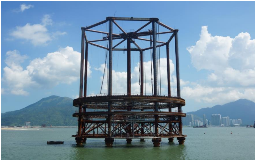
Figure 3. Temporary working platform for sheet piles installation
