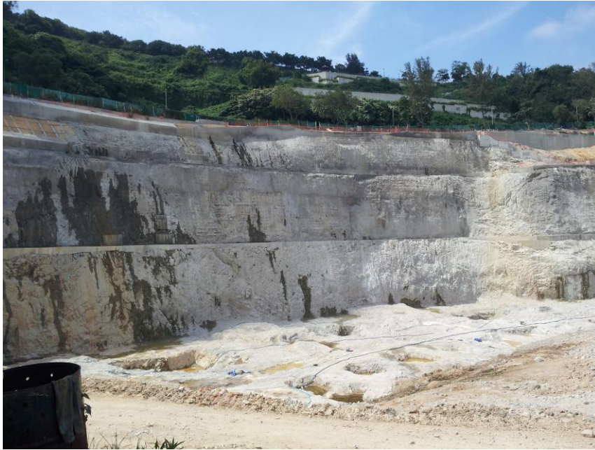
Figure 6 - As-built Condition at Wai Lung Site
