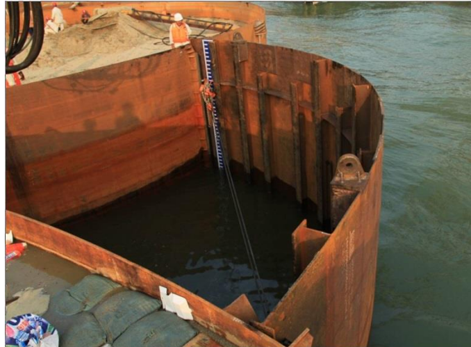
Figure 4. Installation of Arc Cell
