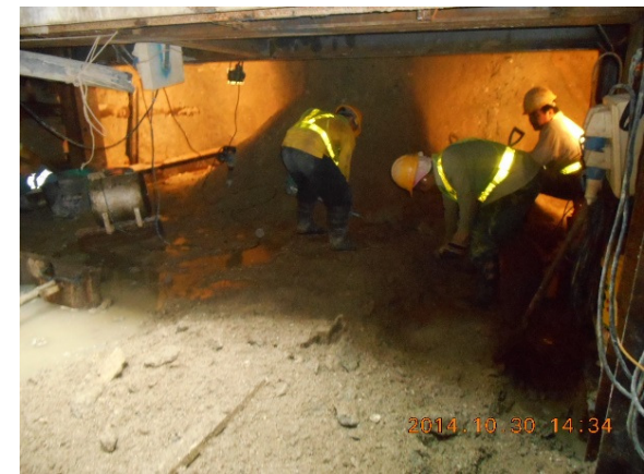
Hand-dug Tunnel Excavation from Working Pit
