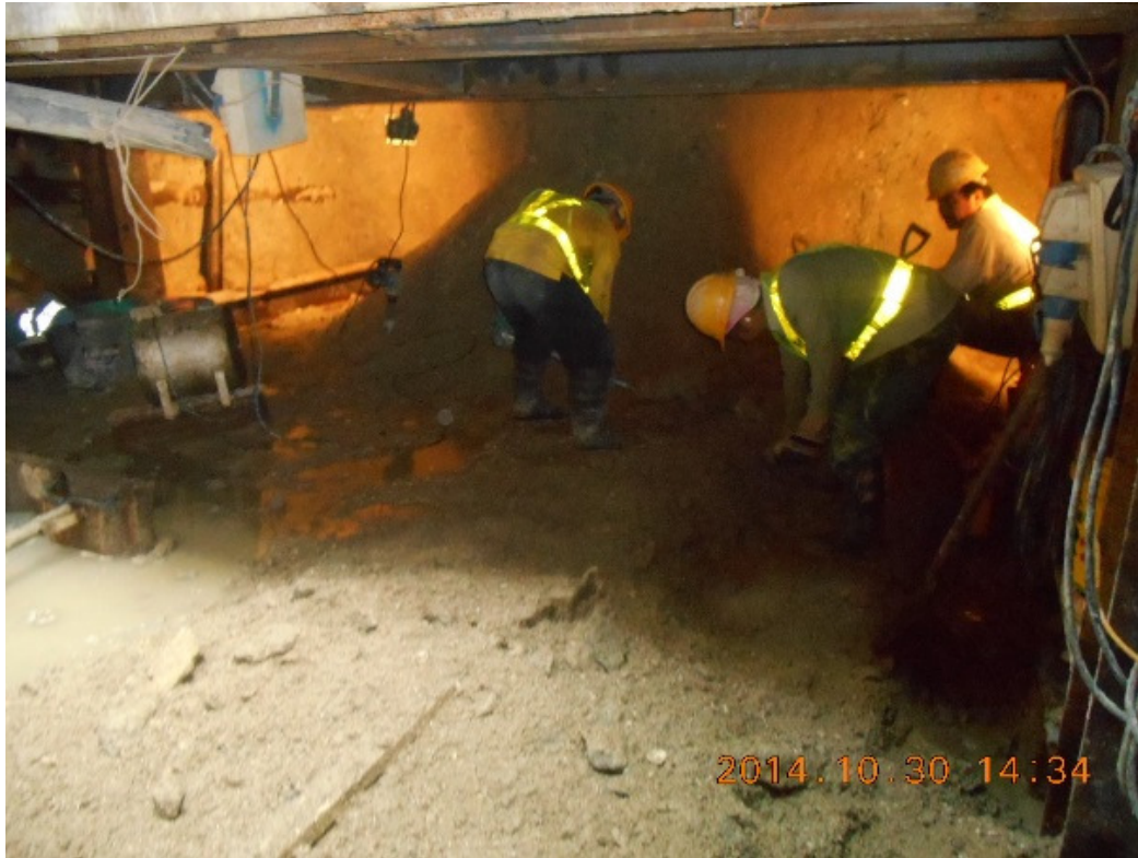
Manual Excavation in Upper Bench of Hand-dug Tunnel
