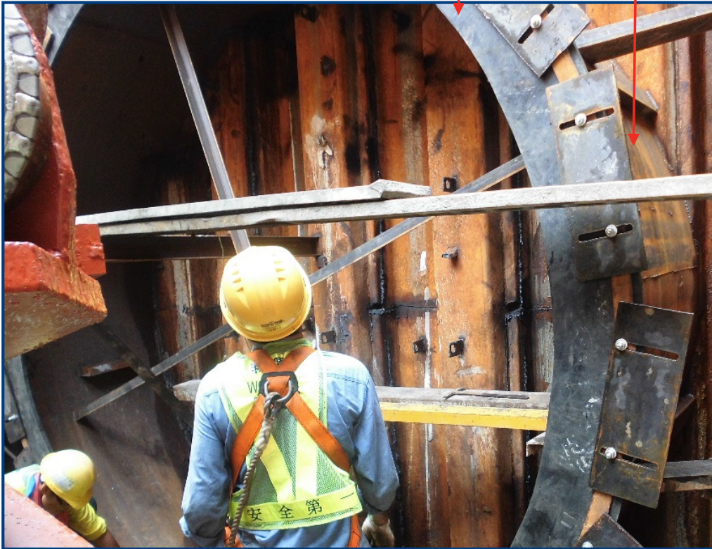
Installation of Entrance Ring
