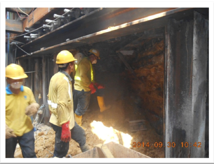
Construction of Hand-dug Caving in Working Pit B-4
