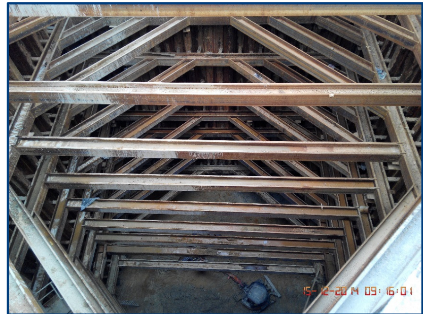
Excavation with Lateral Support for Jacking Pit
