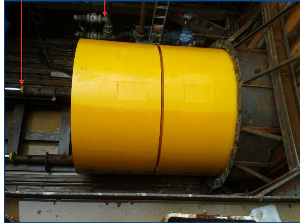
Pushing First Can of TBM to Entrance Ring
