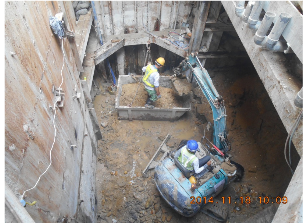
Lower Bench Excavation in Hand-dug Tunnel by Mini-excavator
