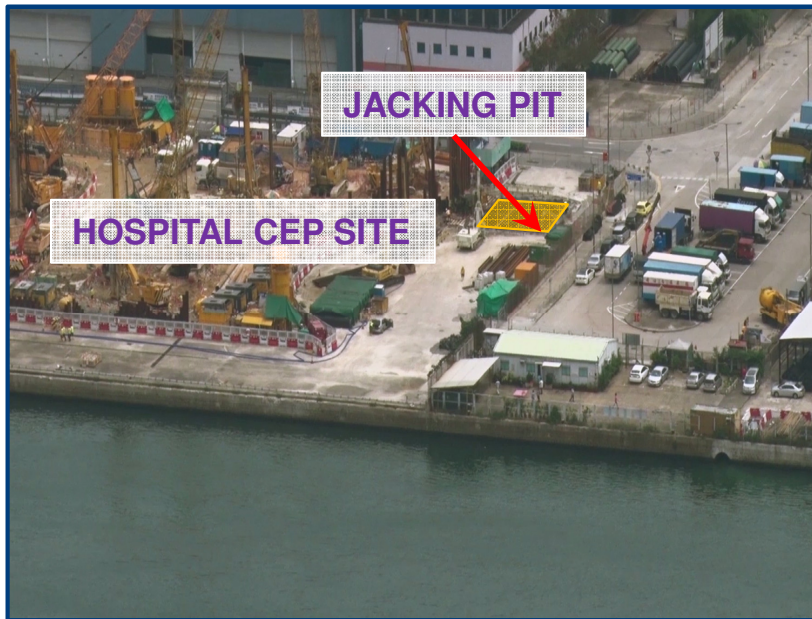
General View of Jacking Pit at Cheung Yip Street and Shing Cheong Road
