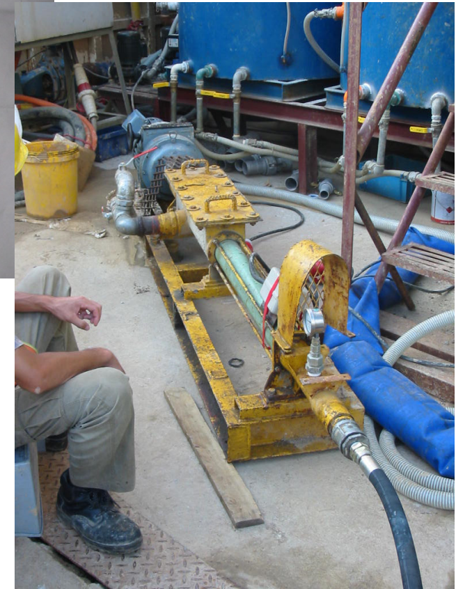
Bentonite Being Pumped to Jacked Pipeline for Lubrication
