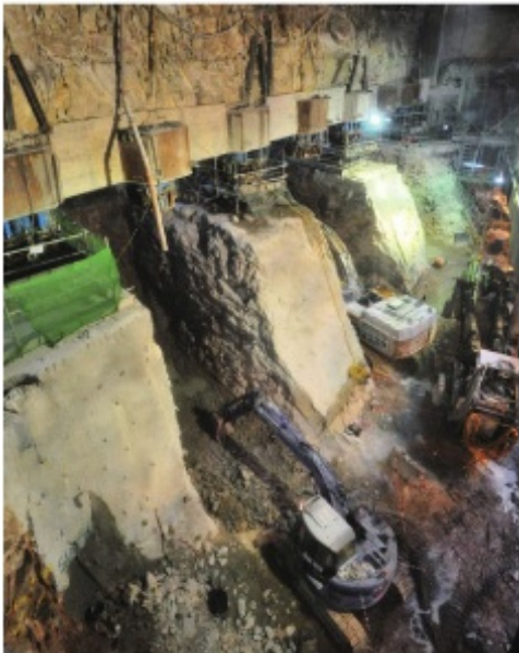
Underpinning structures at Admiralty Station (courtesy of MTR Corporation Ltd)
