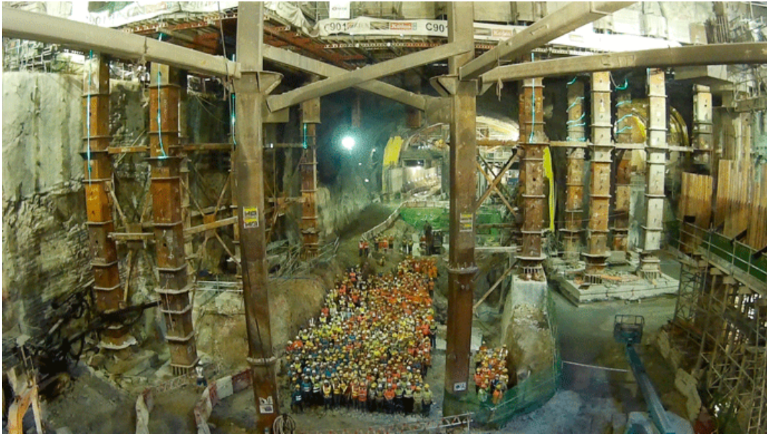
Underpinning structures at Admiralty Station (courtesy of MTR Corporation Ltd)
