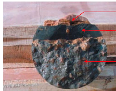
Grout pipe attached to reinforcement cage
