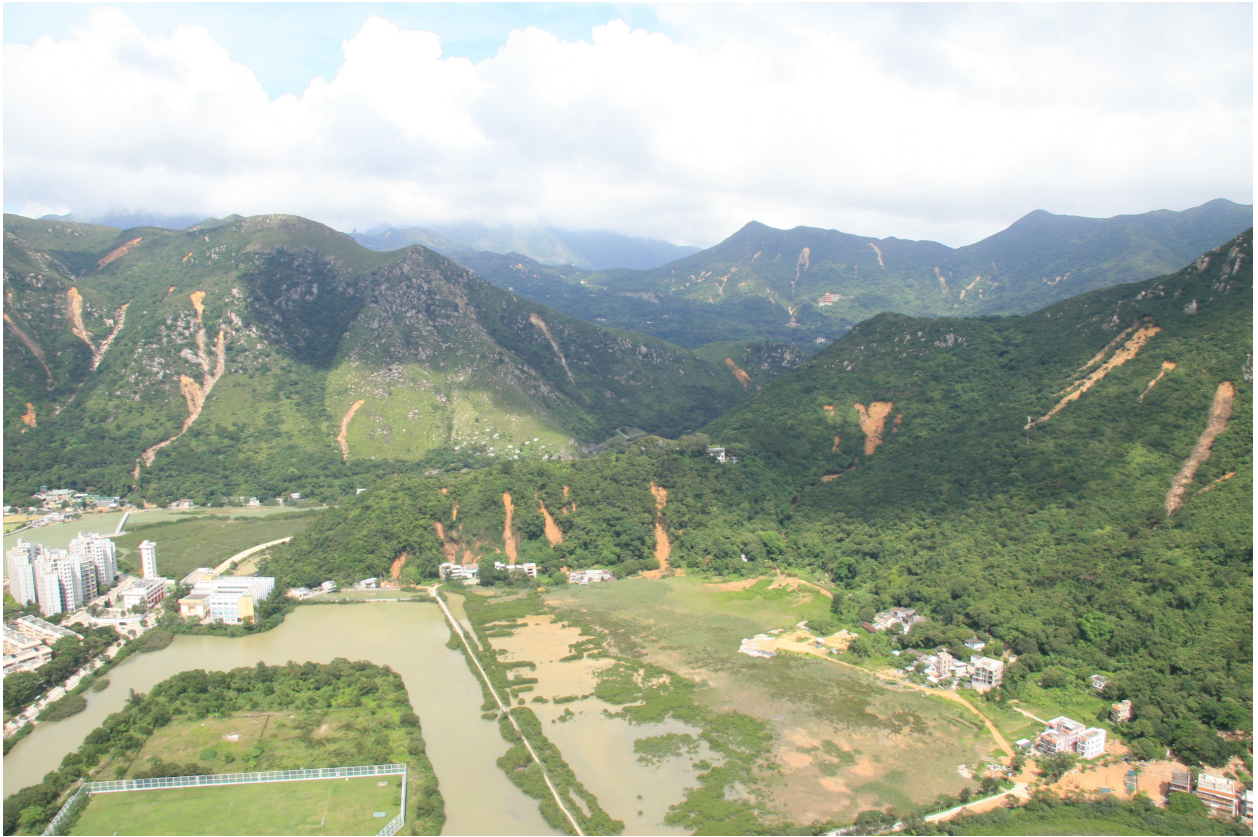
A new framework has been developed for natural terrain hazard studies to meet challenging natural terrain risk management in Hong Kong (courtesy of Geotechnical Engineering Office, HKSAR Government)
