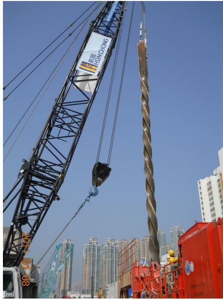
Left: Pile removal by hydraulic jacking (courtesy of Victor Li & Associates Ltd). Right: Pile removal by rotation and wedge method (courtesy of Hsin Chong Construction Group Ltd)
