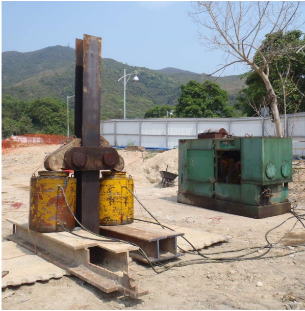
Left: Pile removal by hydraulic jacking (courtesy of Victor Li & Associates Ltd). Right: Pile removal by rotation and wedge method (courtesy of Hsin Chong Construction Group Ltd)
