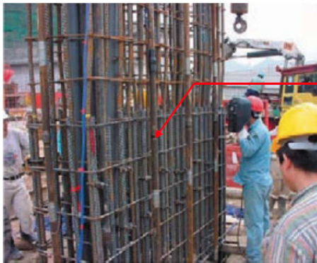
Left: Grout pipes attached to a reinforcement cage. Right: A core sample that shows the cement grout at pile/soil interface achieved through shaft grouting (both courtesy of Ove Arup & Partners Hong Kong Ltd)
