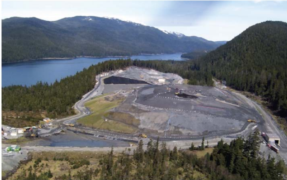
FIGURE 9.1.1 FILTERED TAILINGS FACILITY, GREENS CREEK, ALASKA
