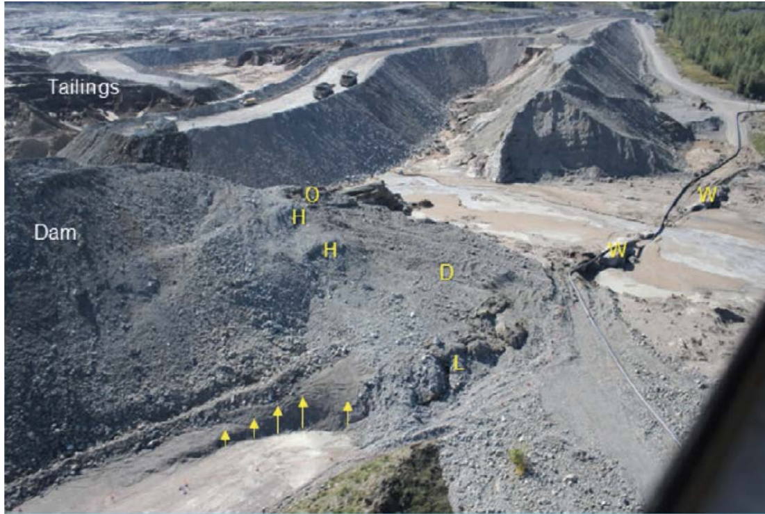
FIGURE 5.1.6: SLIDING-RELATED FEATURES AT RIGHT ABUTMENT (SEPT. 4, 2014 PHOTO)
