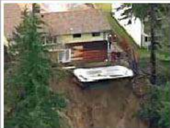
This North Vancouver home's pool hovers on the edge of a cliff which has been drastically eroded by the heavy rains.
