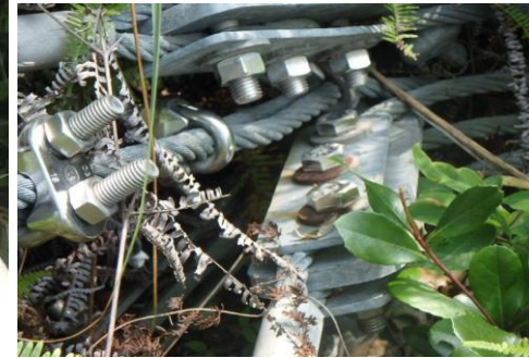
Signs of Minor Rusting at brake element
