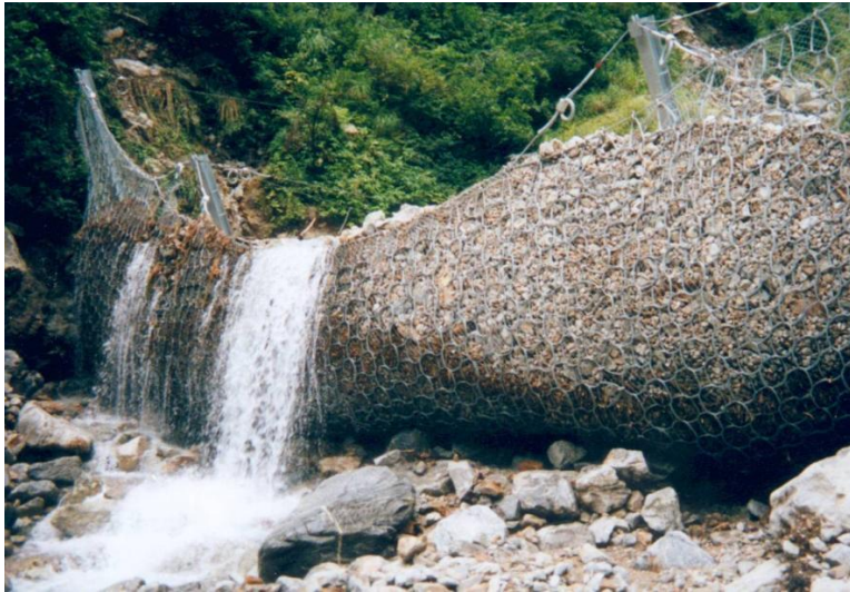
1998: 750 m 3 debris flow in Japan (retained by 1500 kJ rockfall Barrier)
