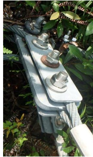
Signs of Minor Rusting at brake element
