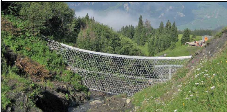
Geobrugg VX Barrier (60-160kPa)
