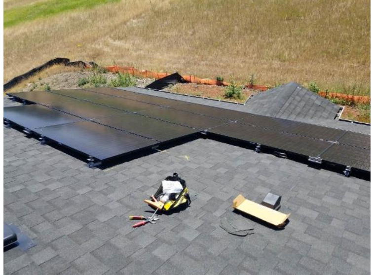
Roof - ARRAY(s) COMPLETED: showing COMPLETE overview of arrays multiple pics and location of soladek (3 pics per array min.) (no close up pics)
