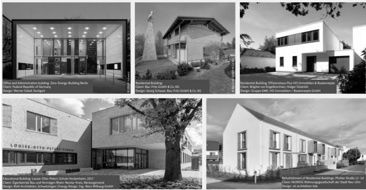
Implementasi Program “ Efficiency House Plus ” di Berlin, Jerman Sumber : Efficiency House Plus in Berlin Report, 2018
