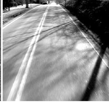
lined two-lane highway
