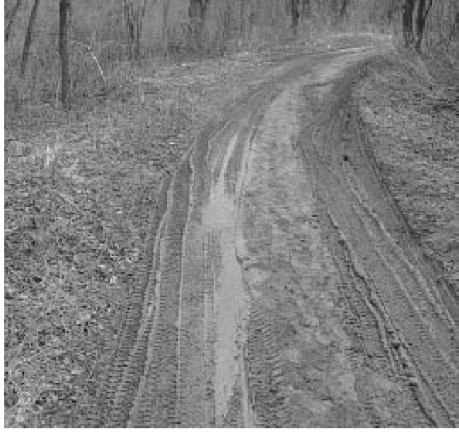
single-lane dirt access road
