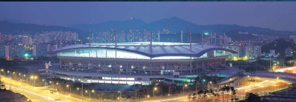
2002 World Cup Main Stadium Seoul, Korea – 2001 Geiger Engineers was the structural engineer for the Seoul World Cup Stadium's
