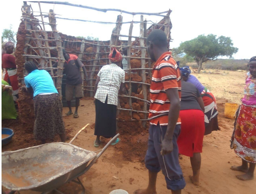
Kithito group doing a house building Mwethia for Mulei.
