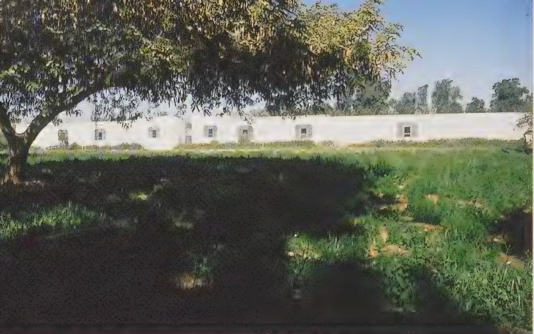
The Atos Company buildings.
